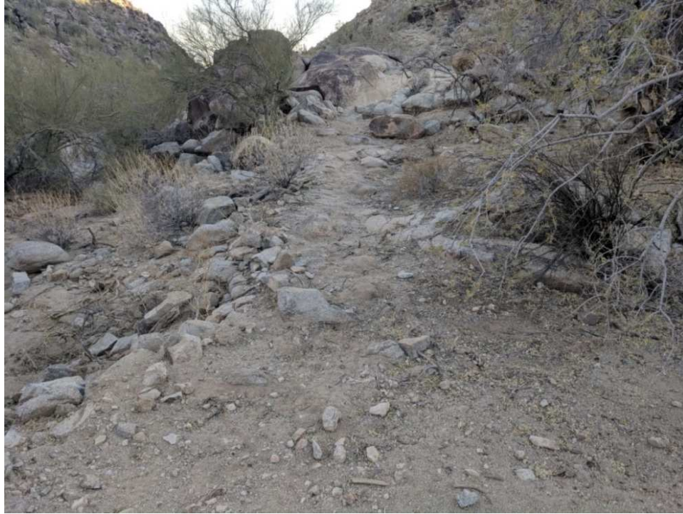
Fig. 10. Damage to trail mitigation, seven days since last visit
