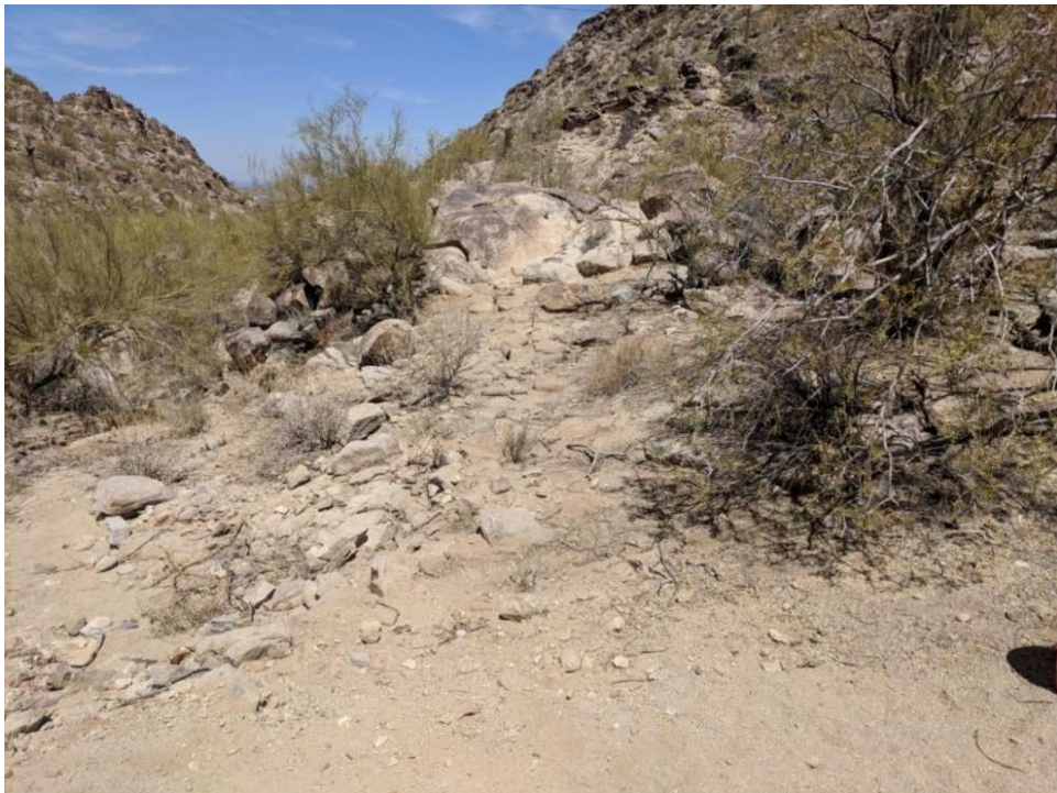
Fig. 4. Completed trail mitigation
