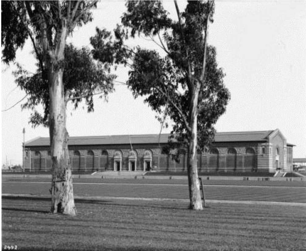
California State Exposition Building, Exposition Park, [s.d.]. California Historical Society Collection, 1860-1960, University of Southern California, Los Angeles, California. Accessed October 11, 2018. http://digitallibrary.usc.edu/cdm/ref/collection/p15799coll65/id/10413 .
