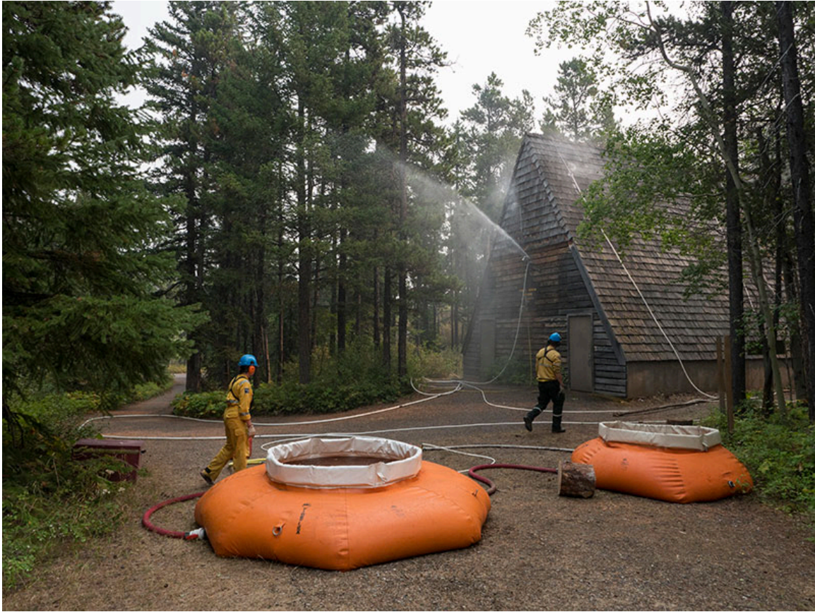
Figure 13 A Parks Canada fire crew testing the sprinkler system at Crandell Theatre, in advance of the arrival of the Kenow Fire. 218
