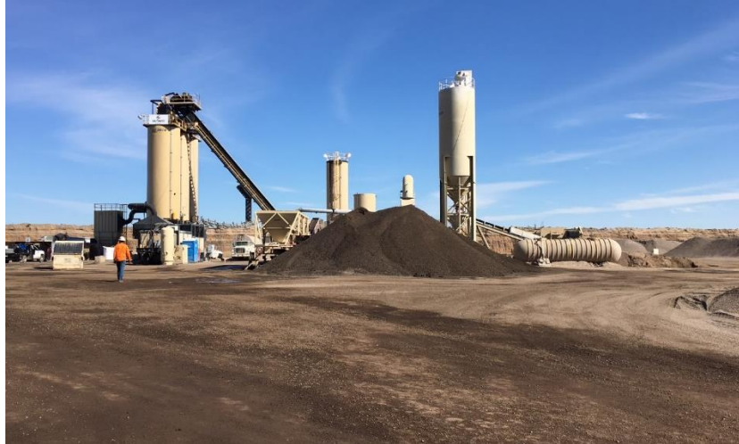
Figure 2-2 RAP processed millings (Southwest Asphalt Plant)
