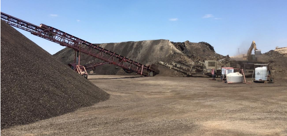
Figure 3-21 Southwest Asphalt plant RAP processing.
