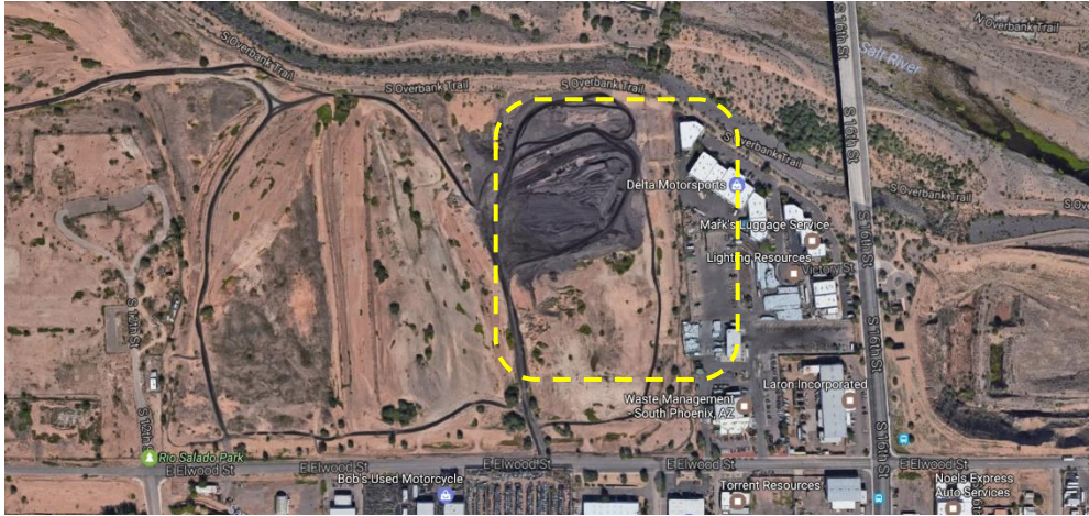
Figure 3-3 General sight of the stockpile site in Del Rio Landfill
