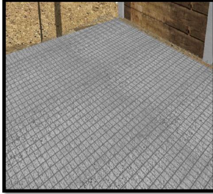
Figure: Reinforcing Steel placed
