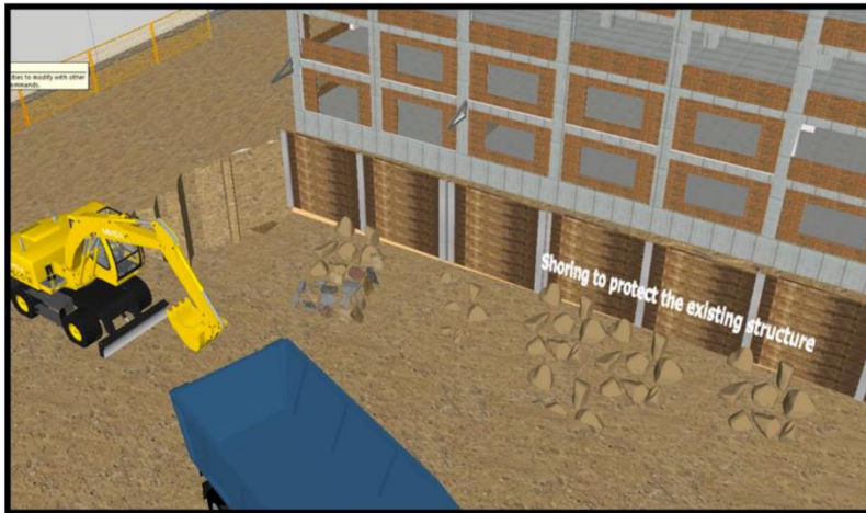
Figure 6. Shoring to protect the existing structure
