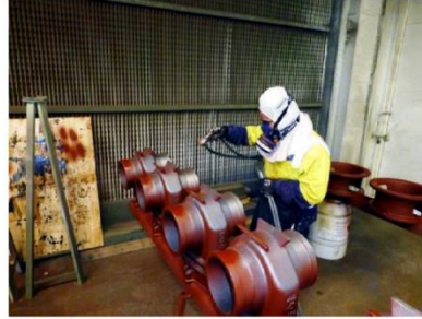
Figure 15 (b). Painting before installation
