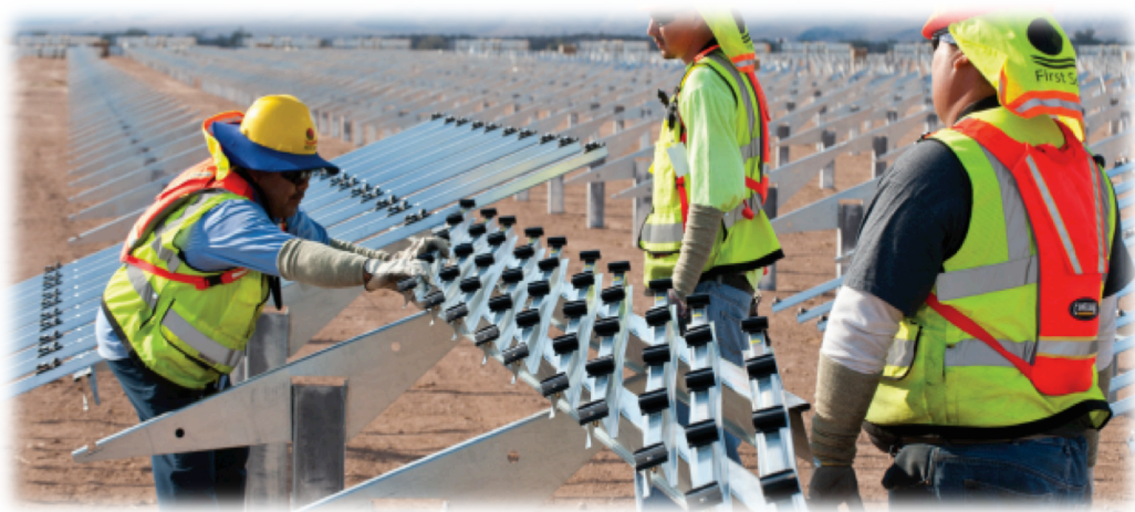
Figure 4. First Solar Driven Posts (First Solar Procurement and Construction Management, 2017)
