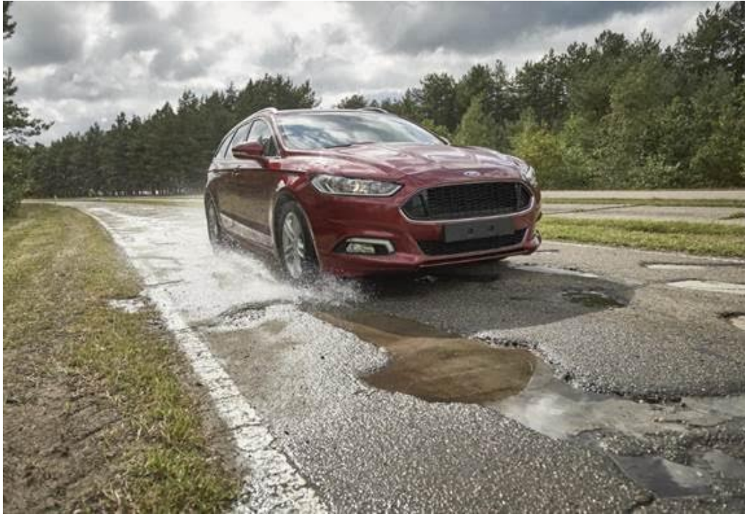
Figure 1.1 Poor pavement condition may contribute to driver distraction, substandard vehicle operation and accidents
