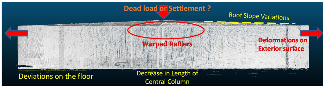
Figure 4. Spatial changes of a steel water tank
