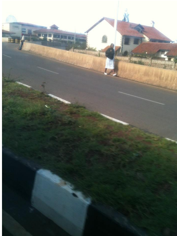
Figure 3.9 A Pedestrian Walking on a Newly Renovated Motorway
