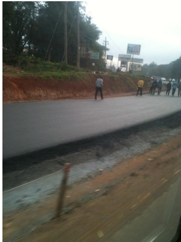
Figure 3.8 A New Highway under Construction
