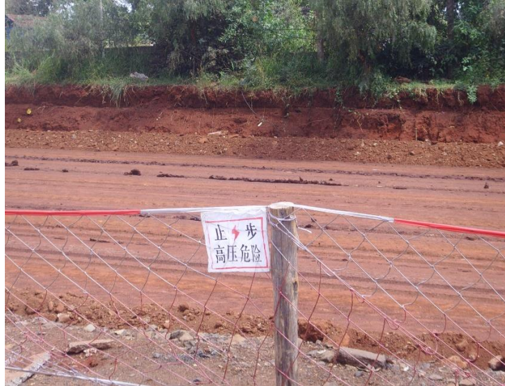
Figure 1.4 A Danger Sign Written in Chinese at a Road Construction Site
