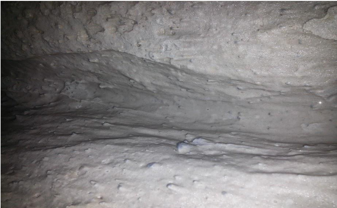
Figure 72: Cement nodules within the concrete. Concrete mixes of the same sand: cement ratio showed no significant change in tensile strength with or without these features.
