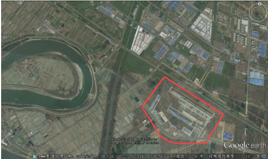
Figure 4.2.10: Wuhan Railway Container Center Terminal (Source: Photo by the Author)
