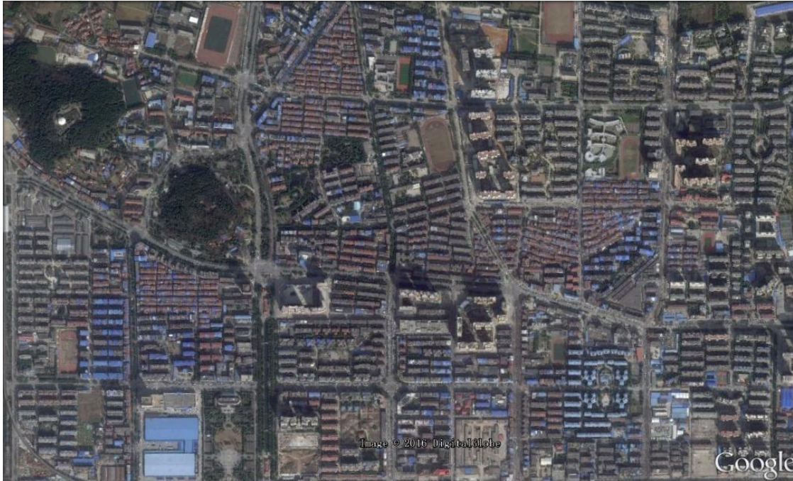
Figure 4.1.4: The Old Town of Dongxihu District (Source: Google Earth, image date: 2016)
