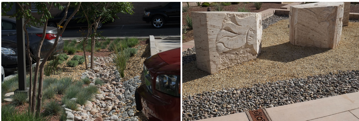
Fig. 5. Bioswale in Parking Lot (Left) and Infiltration Rock Garden in Entry Plaza (Right) at Domenici Courthouse in Albuquerque, NM USA.
