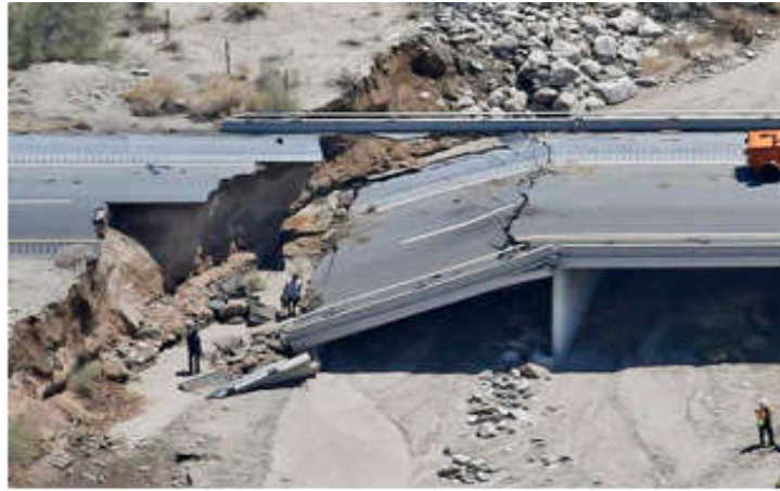
Figure 1. Damage Examples of Aircraft Structural Components; (A) Aloha Airlines Flight 243; (B) Southwest Airlines Flight 812 (Courtesy: Google Image); And (C) Highway Bridge Collapse Due to Flash Flood and Scour (Courtesy: NPR News)
