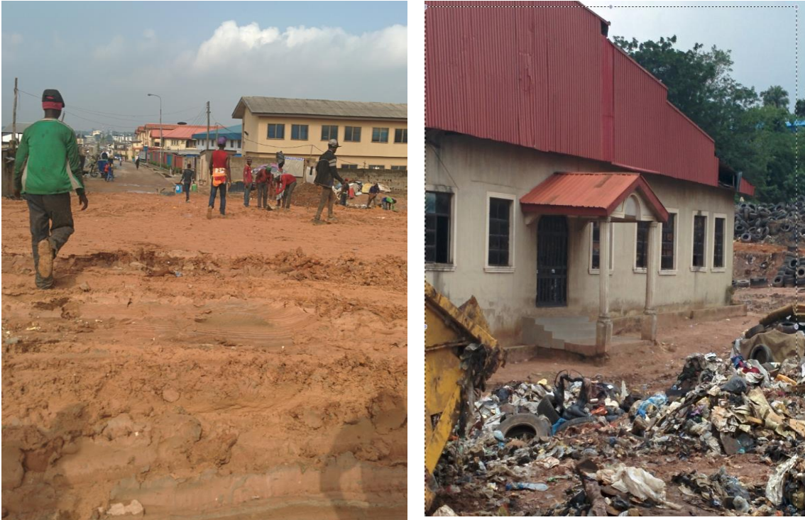
Pictures taken during field survey at Olushosun landfill in Lagos
