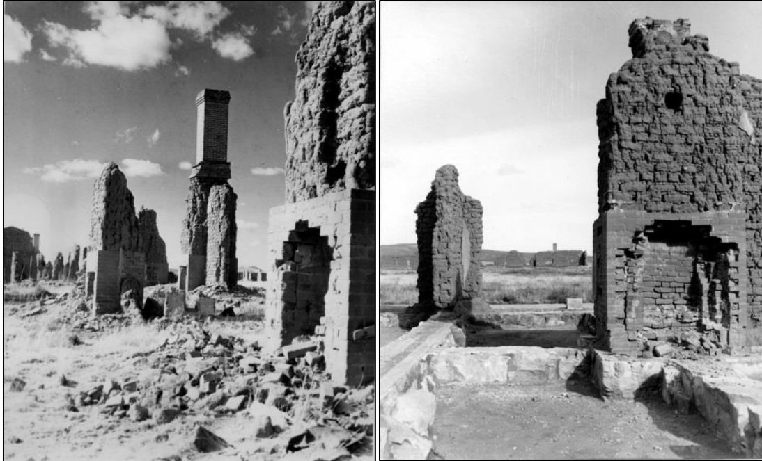
Figure 25: Officer's Quarters, c.1955 (left) and c.1960. Note removal of infill material around foundations. (Source: Fort Union National Monument Photo Files)
