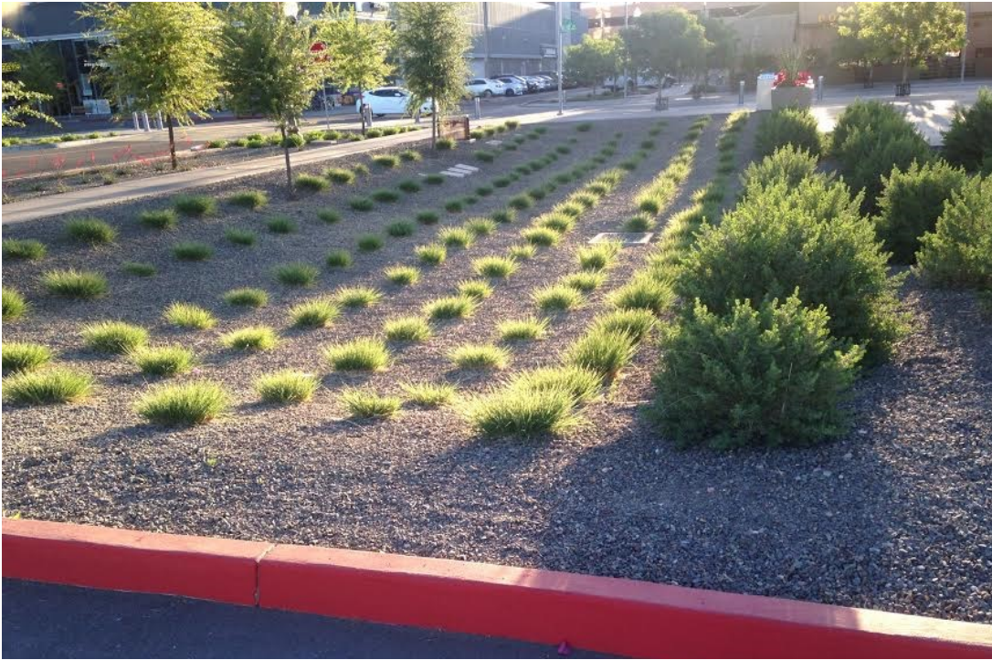
Figure 20. Bioretention Basin Installed at CAVC Development. Photos: Mason Lacy
