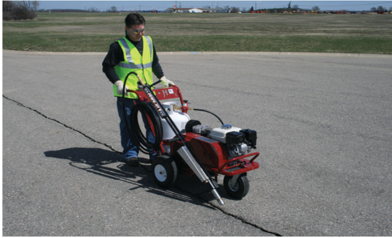
Figure 2-9: Snapshot of Crack Cleaning Using Air blaster [6]
