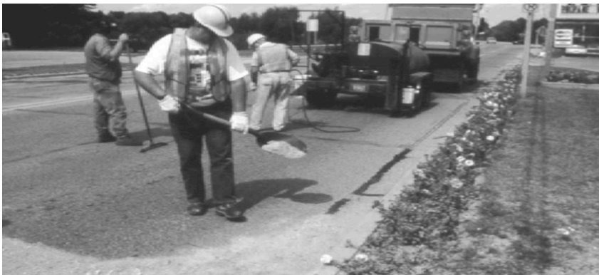
Figure 2-11: Blotting By Pouring Clean Sand Over Sealed Crack [10]
