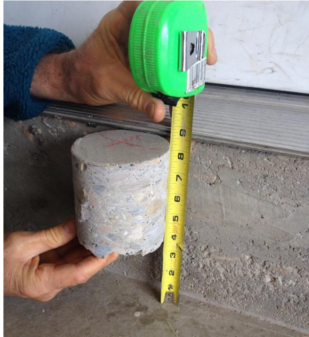
Figure A.5. Photo of a slab core taken during the installation of internal subsurface monitoring locations. The photo is shown next to the step from the garage to inside of the house.
