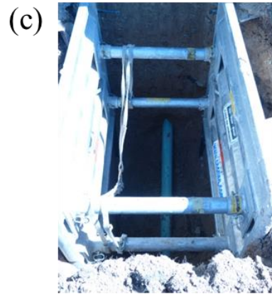
Figure A.6. (a) Schematic showing the location of the lateral pipe and land drain system relative to the front of the study house; photos (b) of the excavation process to uncover the lateral pipe and (c) the uncovered lateral pipe.
