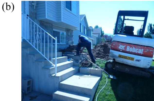
Figure A.6. (a) Schematic showing the location of the lateral pipe and land drain system relative to the front of the study house; photos (b) of the excavation process to uncover the lateral pipe and (c) the uncovered lateral pipe.
