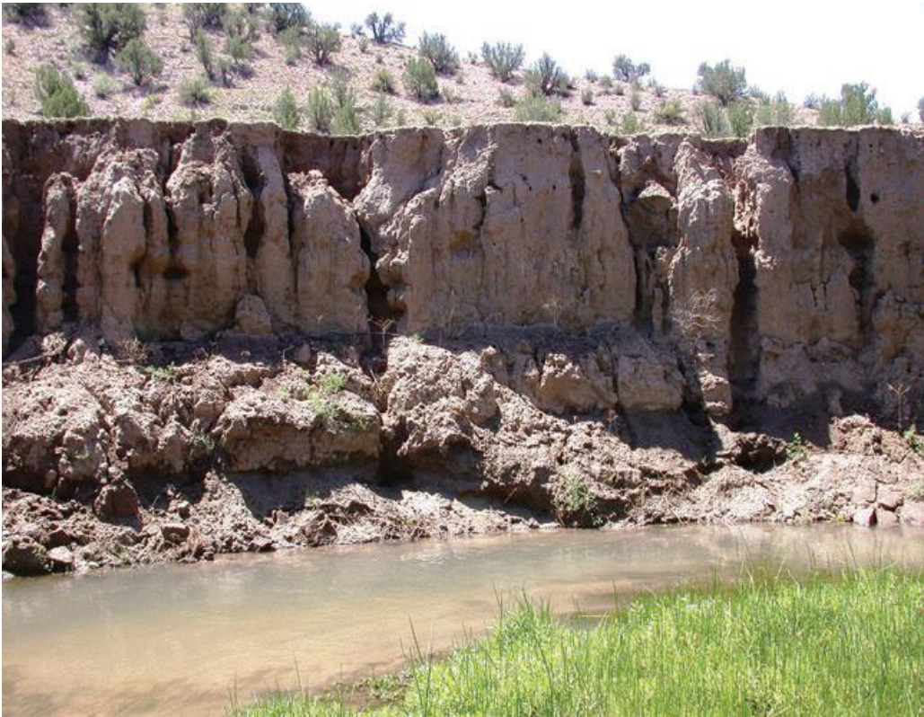
Figure 13. Arroyo cut near Morgan's Ranch showing the Verde River ca. 4 meters below its previous level (Photo courtesy of Neary et al. 2012) .
