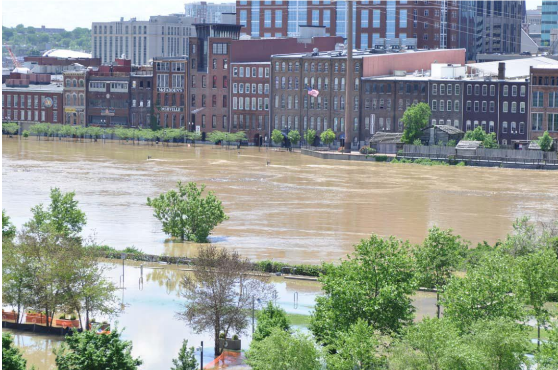
Figure 2.19: Flooding along First Avenue on the Cumberland River near Downtown Nashville ( Source: USACE, 2012 )
