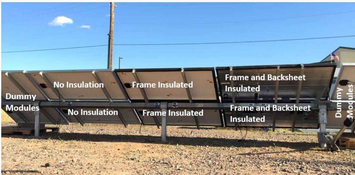
Figure 17. Modules mounted on open rack fixed at 33°S – Back View
