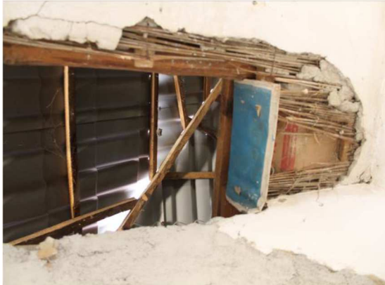
c. Roof detail from inside
