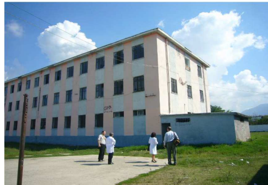
b. Type 3 Building Rear
