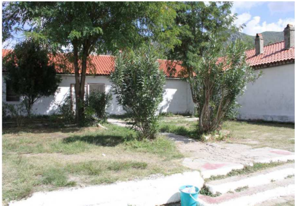
a. Existing School Building
