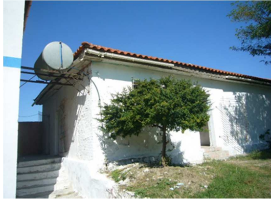
b. Roof Exterior
