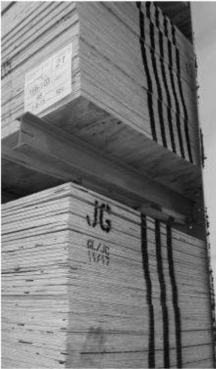
Figure 8. End stripes on sheet goods indicating the thickness of the material.
