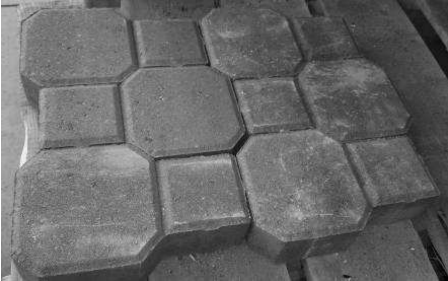
Figure 7. Pavers laid out to determine the quantity in a square foot.
