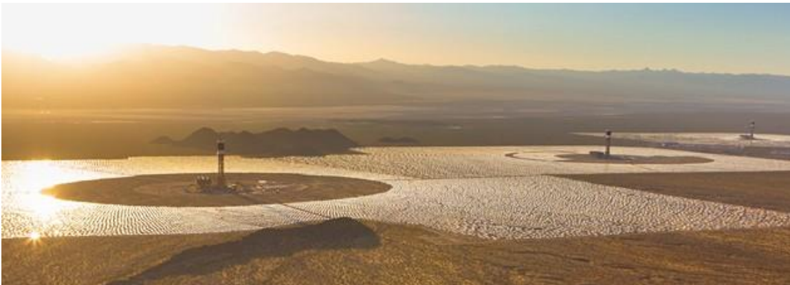
Figure 23. The Ivanpah Solar Electric Generating System (2014). Source: BrightSource Energy.
