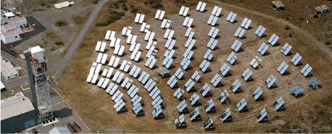
Figure 6. The CRS Tower Plant in Spain, 1981. Source: Plataforma Solar de Almeria website. Used with permission. 27
