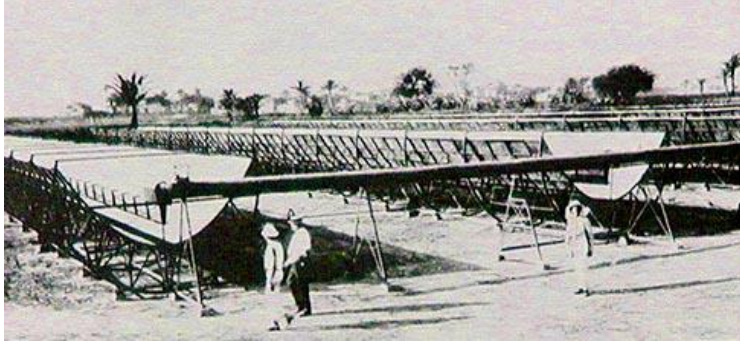
Figure 4. Frank Shuman's Solar Engine I: Meadi, Egypt, 1909 (Suburb of Cairo). From PESWiki (public domain) 26
