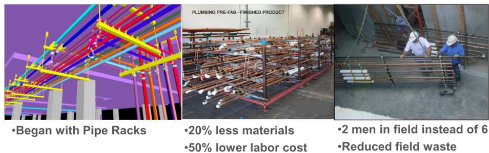
Figure 7. Productivity Improvements in a BIM to Fabrication Workflow for Pipe Racks. Reprinted from Global Industry Trends with Building Information Modeling by S.A. Jones, 2013.
