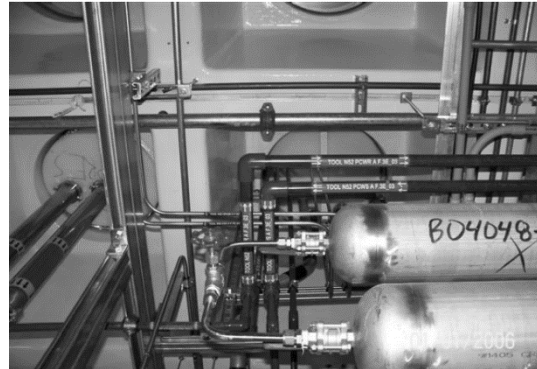
View of the Popouts in the waffle slab (viewed from the sub-fab)
