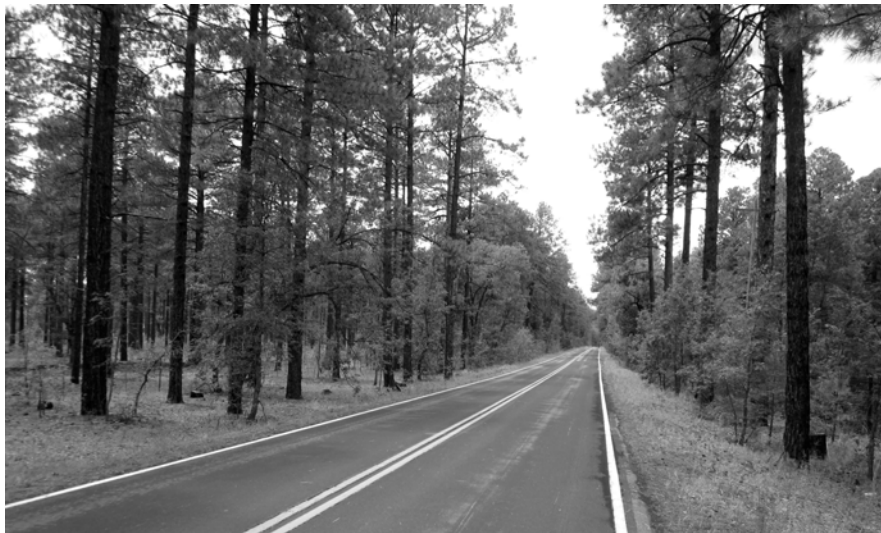
Figure 20: A Road Divides: Pinetop-Lakeside & The White Mountain Apache Reservation
