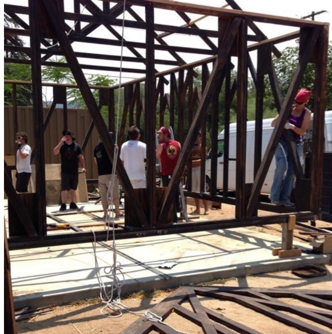
Photograph 8. Building Church Trap. Photo by author.
