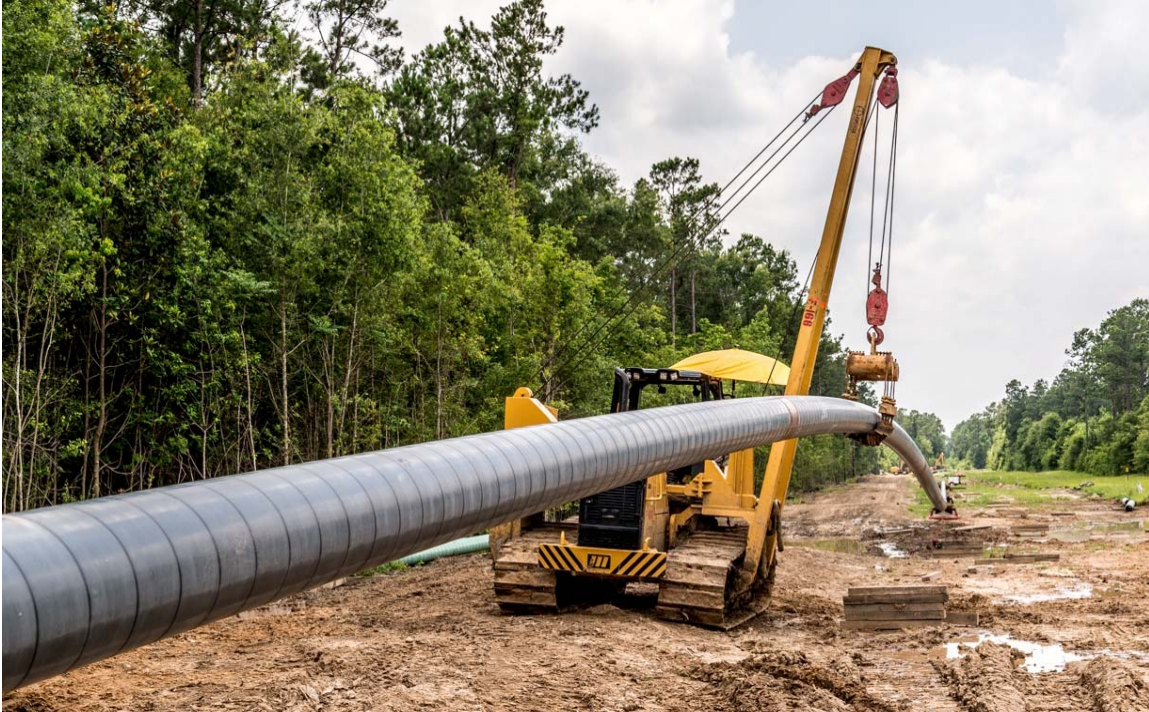
Figure 5.49: Product Pipe During Pullback (Ranger)
