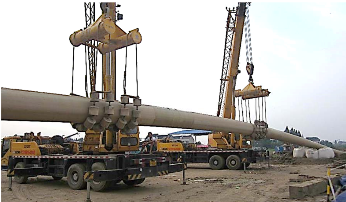
Figure 5.13: Pipe Stringing Operations During Final Pullback
