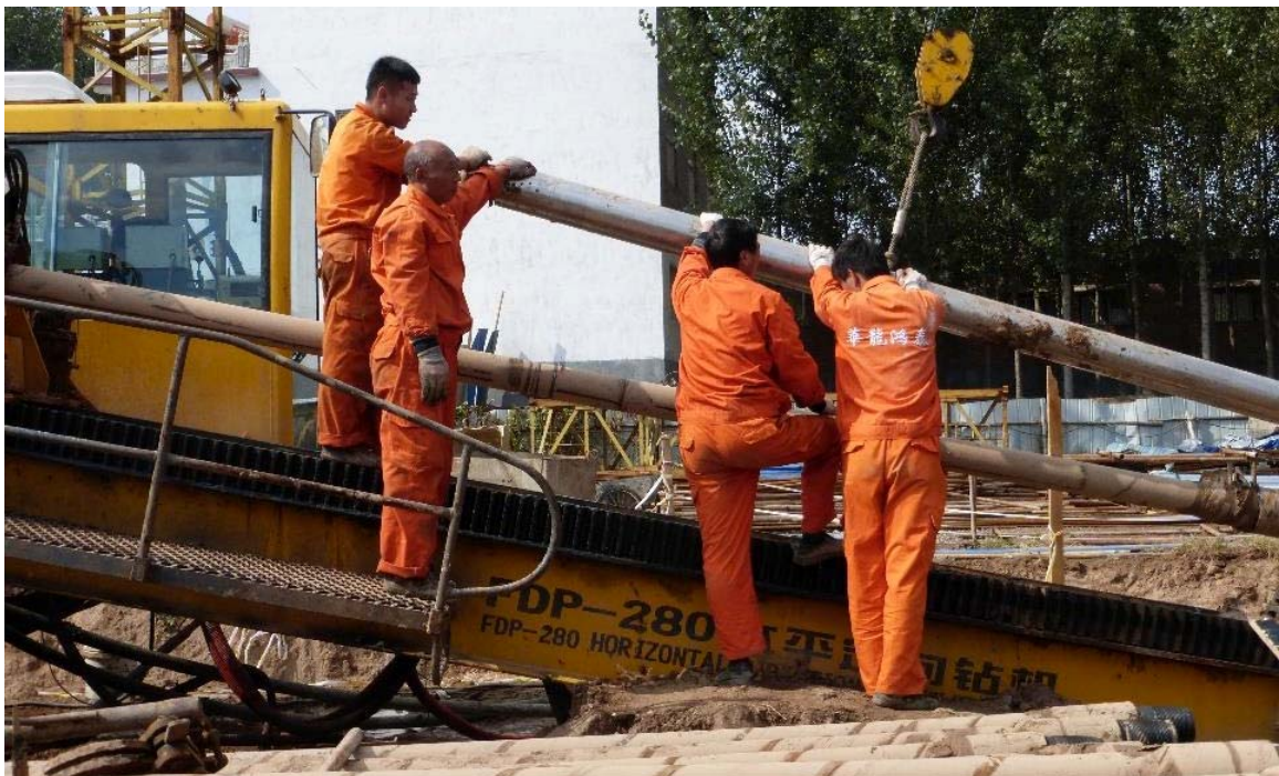
Figure 1.2: Chinese Workers Working of Horizontal Directional Drill Rig
