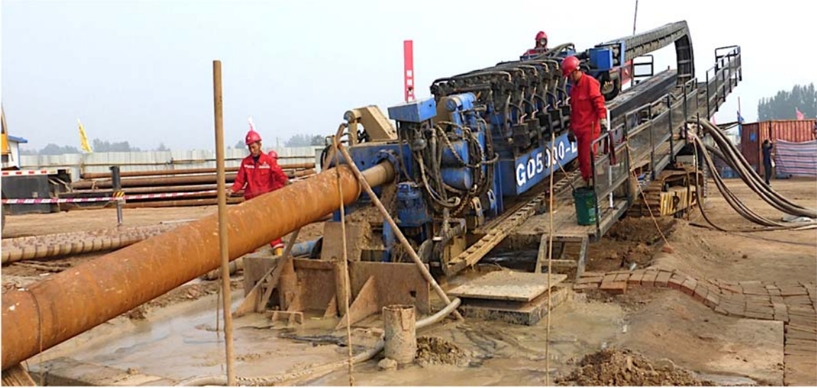
Figure 5.17: Main Rig - Shanghai Goodeng GD5000-LL Drill Rig
