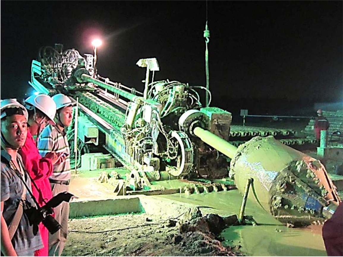
Figure 5.14: Nighttime Pullback Operations
