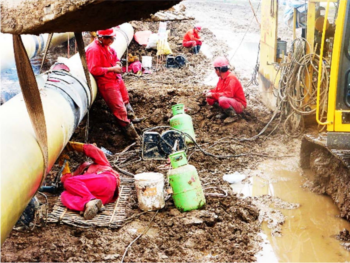
Figure 6.16: Onsite Welding Operations
