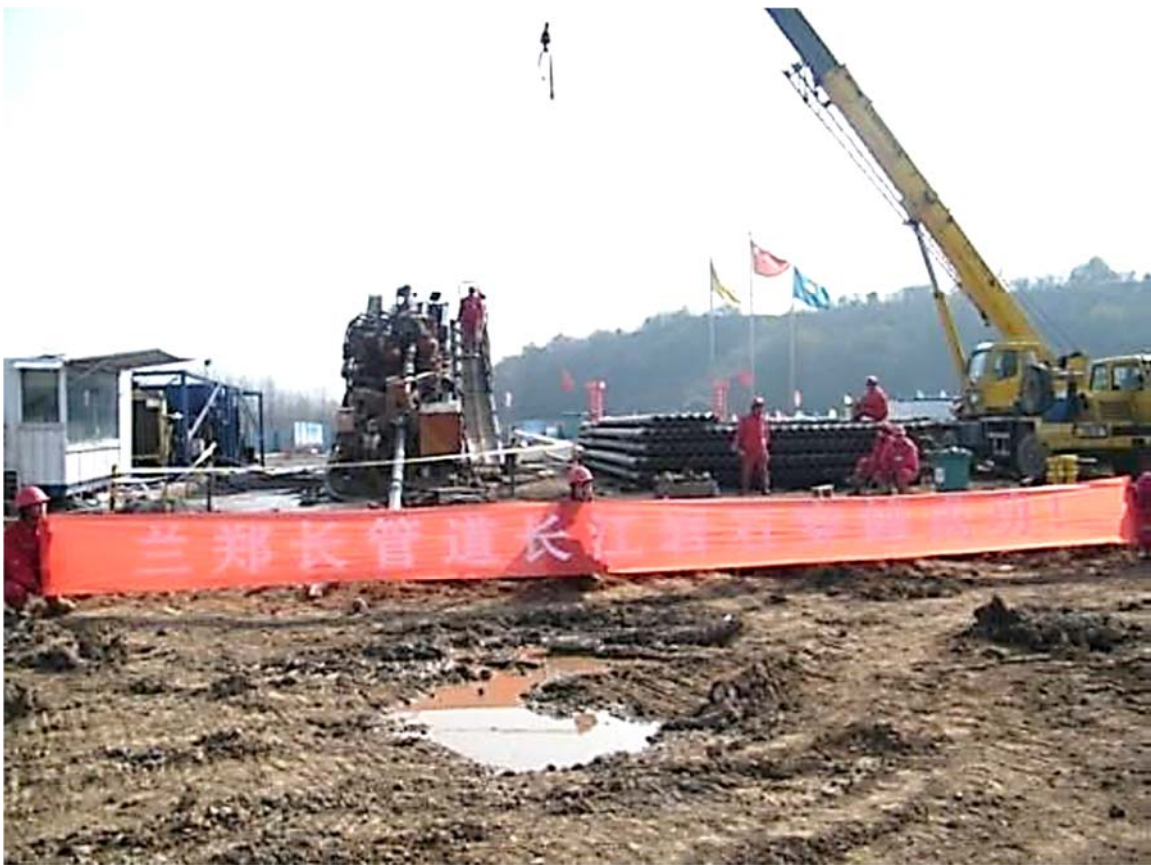
Figure 5.35: Successful Pipeline Pullback (Li et al, 2013)
