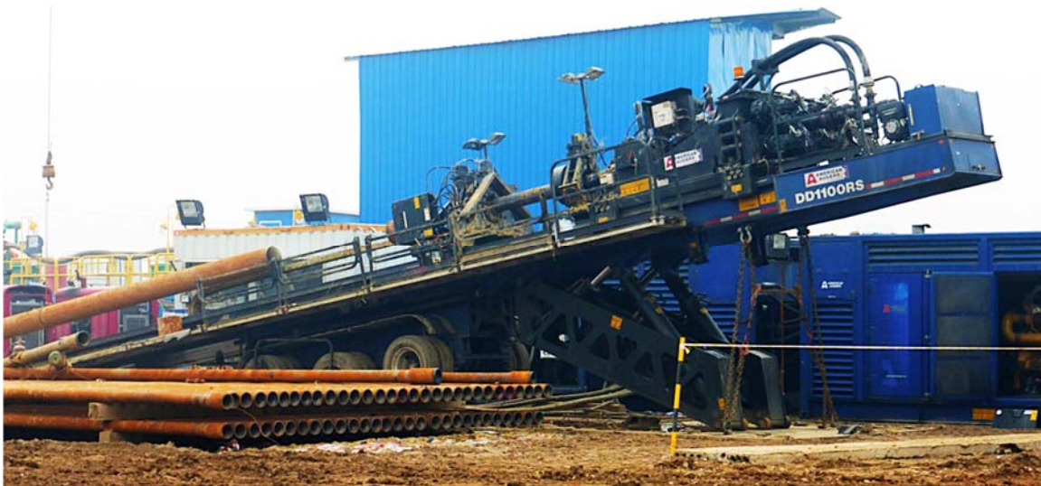
Figure 5.9: Main Rig - American Augers® DD-1100RS Drill Rig
