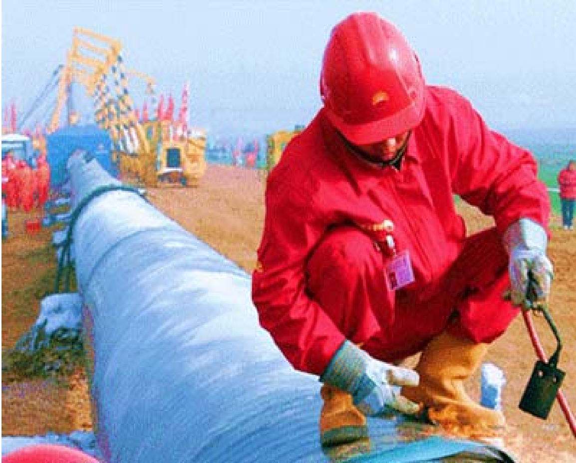
Figure 3.2: CNPC Inspector on HDD Pipeline Installation ( www.cnpc.com.cn/en )
