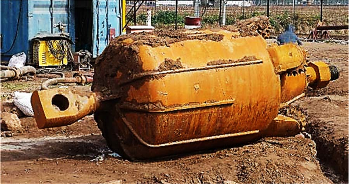
Figure 6.22: Rusted Barrel Reamer – China
