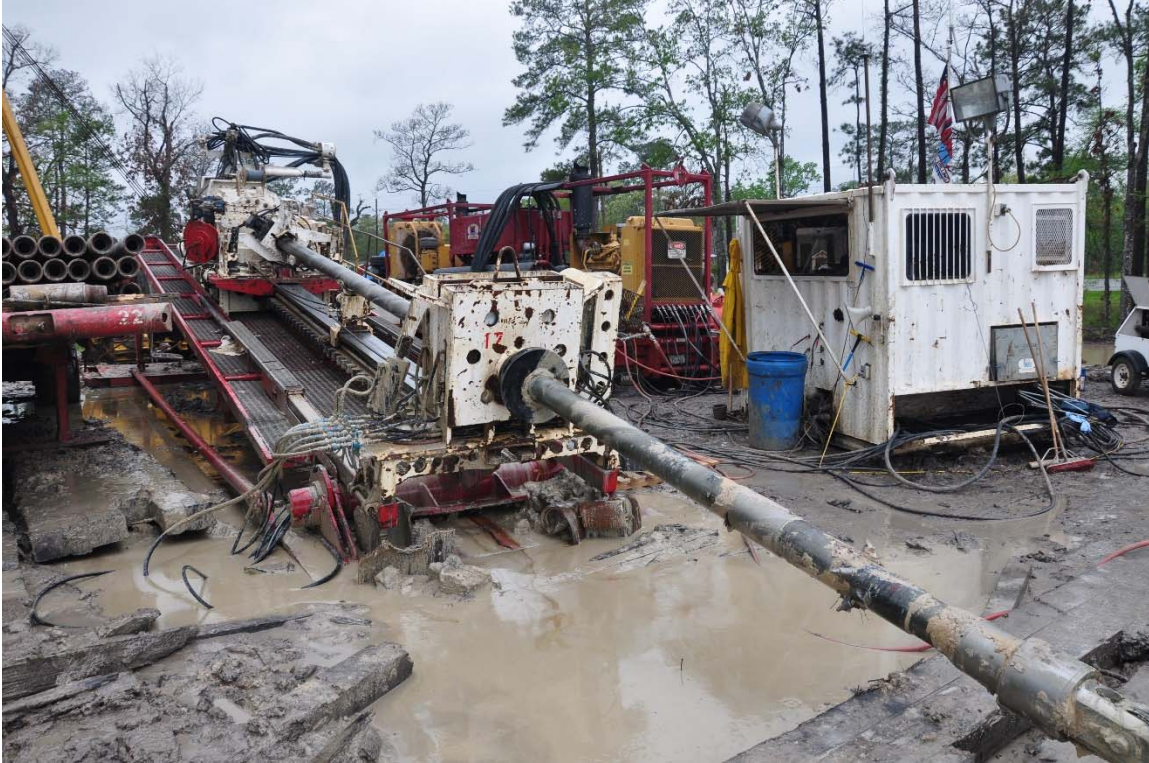
Figure 5.44: LDD 750 Drill Rig (Laney 2013)
