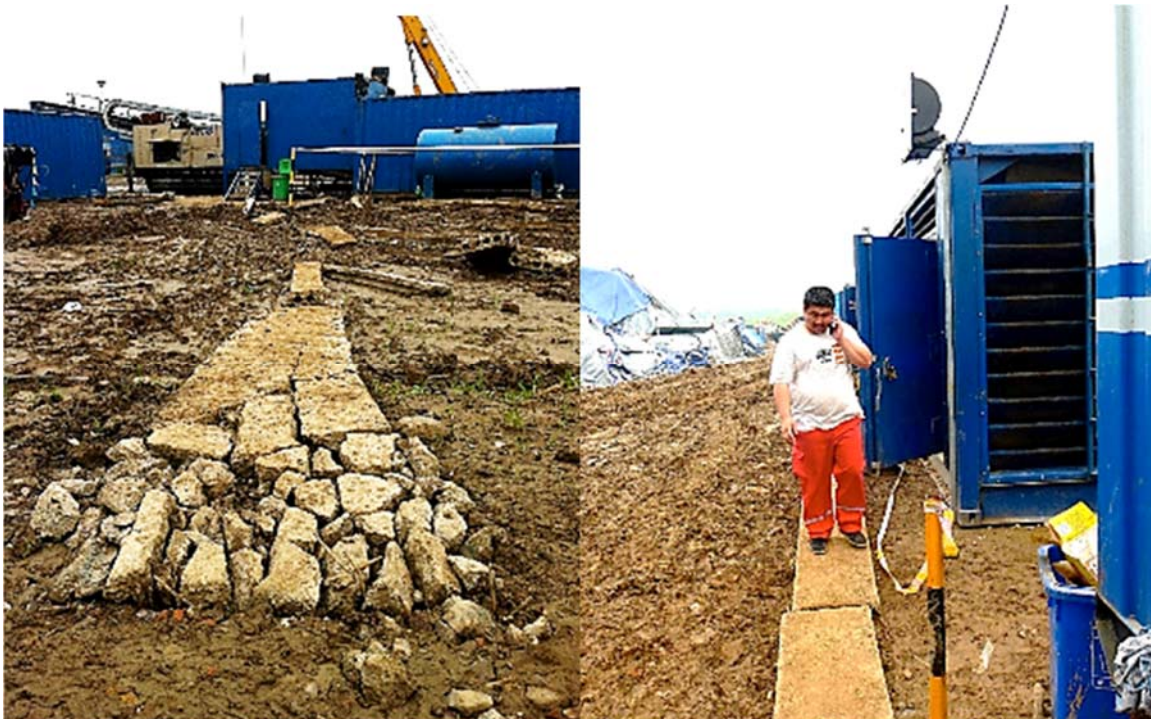
Figure 6.14: Preformed Concrete Panels Used for Walking Paths
