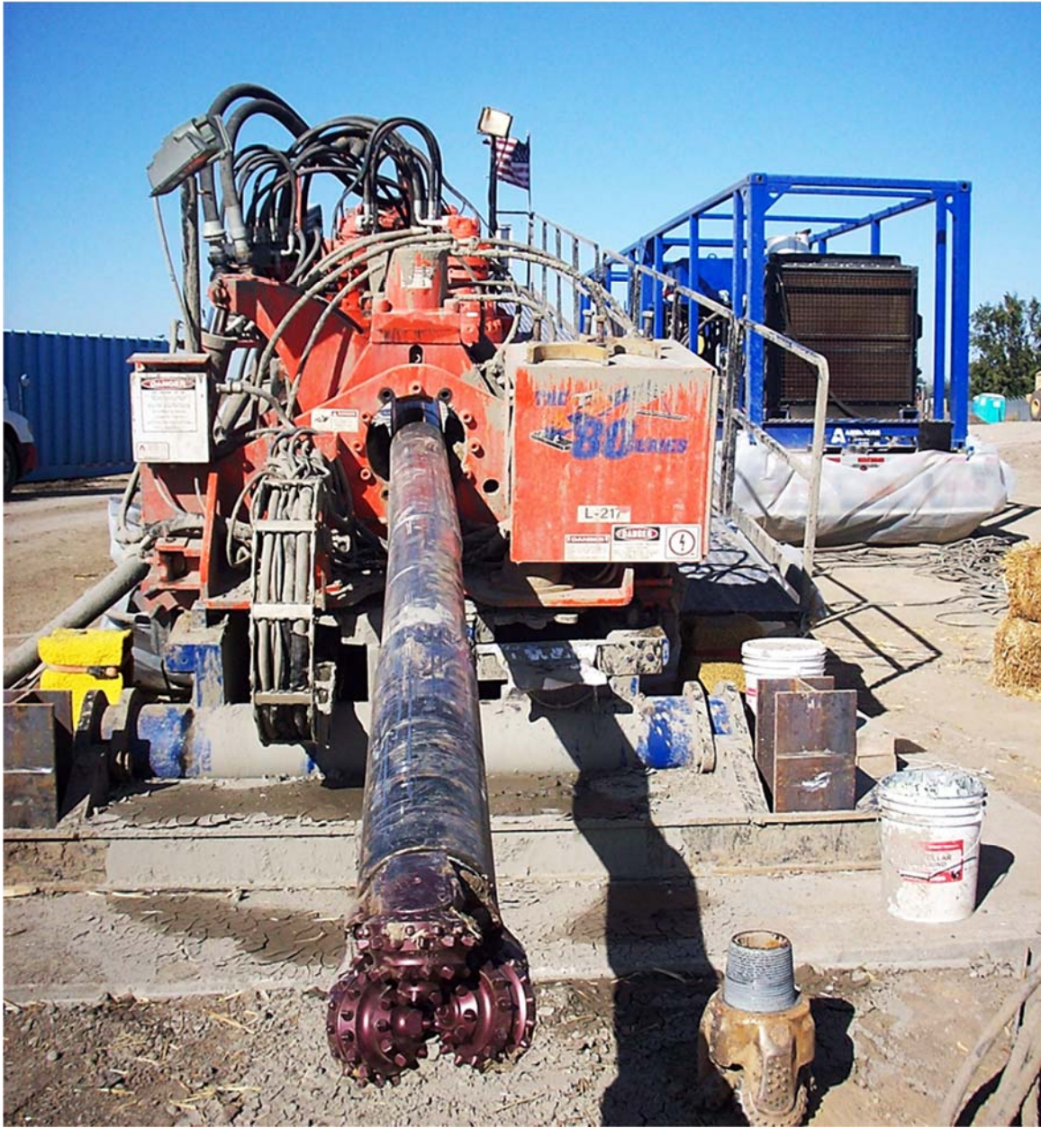
Figure 5.53: Main Drill Rig
