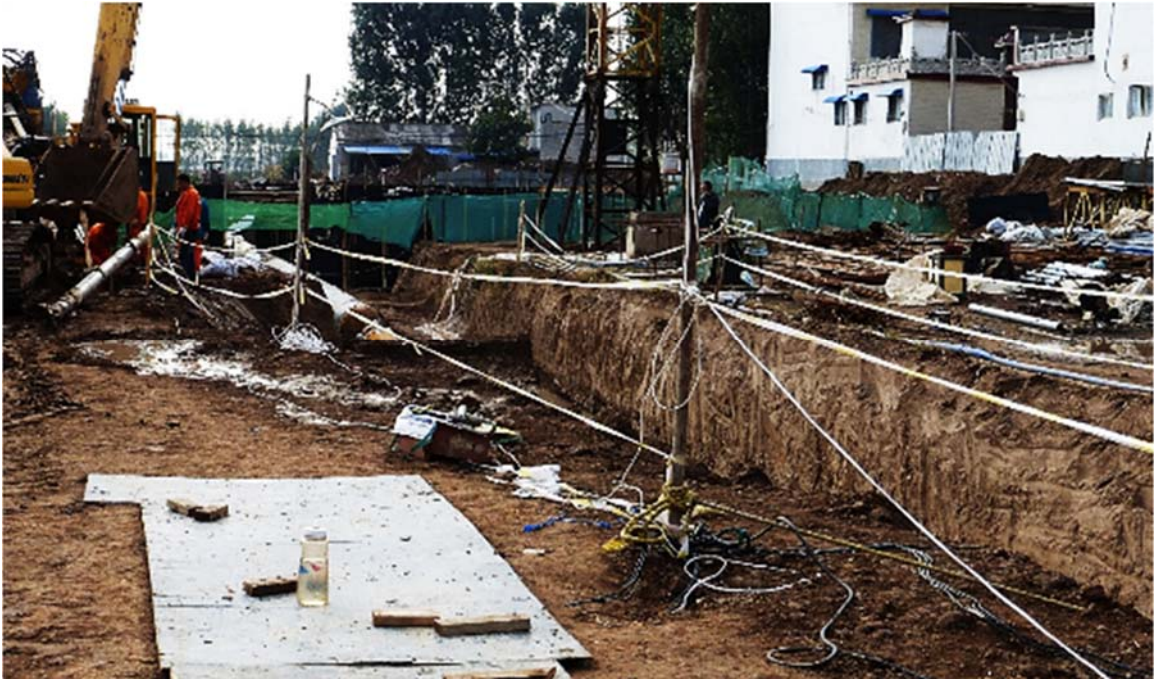
Figure 6.34: Trenching Adjacent to Tower Crane
