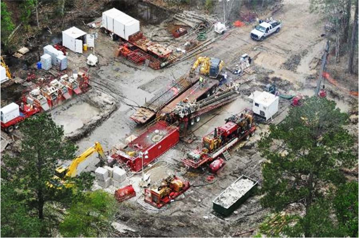
Figure 6.12: Application of Timber Matting for Total Project Drill Area
