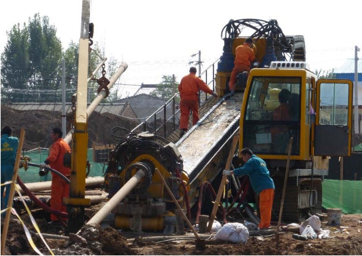
Figure 5.23: Auxiliary Drill Rig Located on Exit Side
