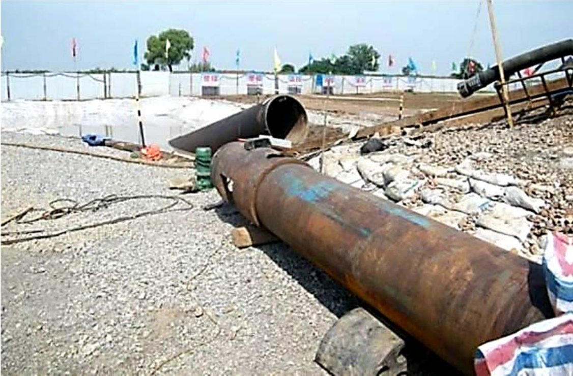
Figure 5.30: Casing Tamping Field on the South Bank (Li et al, 2013)
