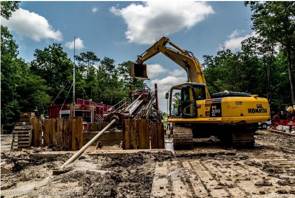
Figure 5.50: Successful Pipeline Pullback (Ranger)
