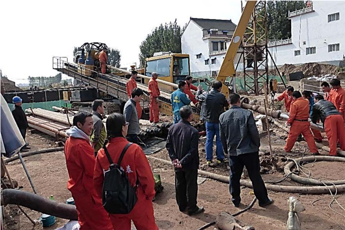
Figure 5.27: Onsite Workers During Recovery Operations
