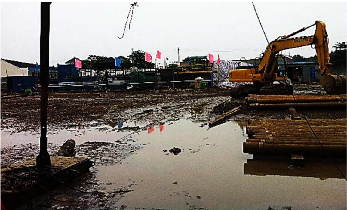
Figure 6.12: Application of Timber Matting for Total Project Drill Area
