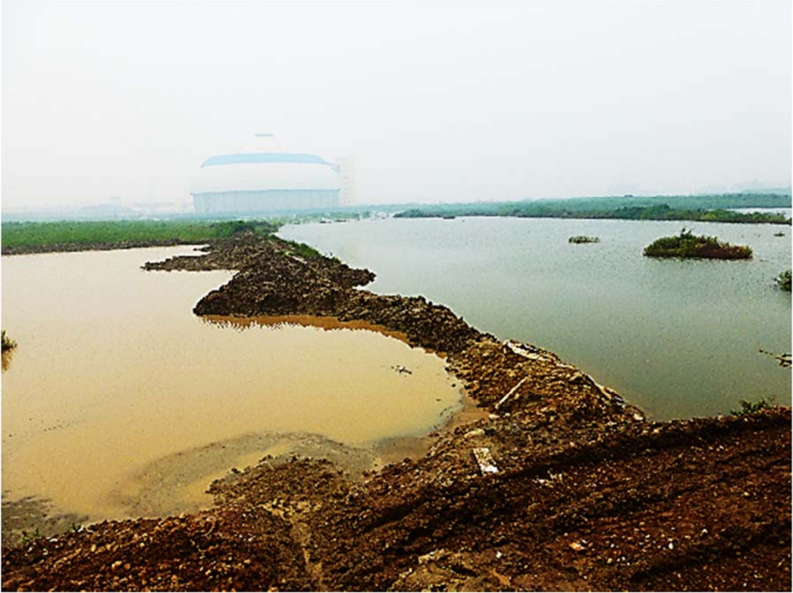
Figure 6.26: Cuttings Retention Ponding Systems (Example 1)
