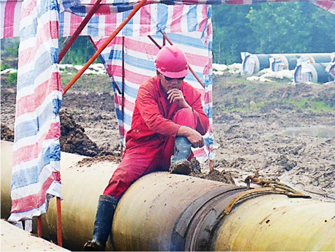
Figure 6.37: Onsite Continuous Welding Inspections
