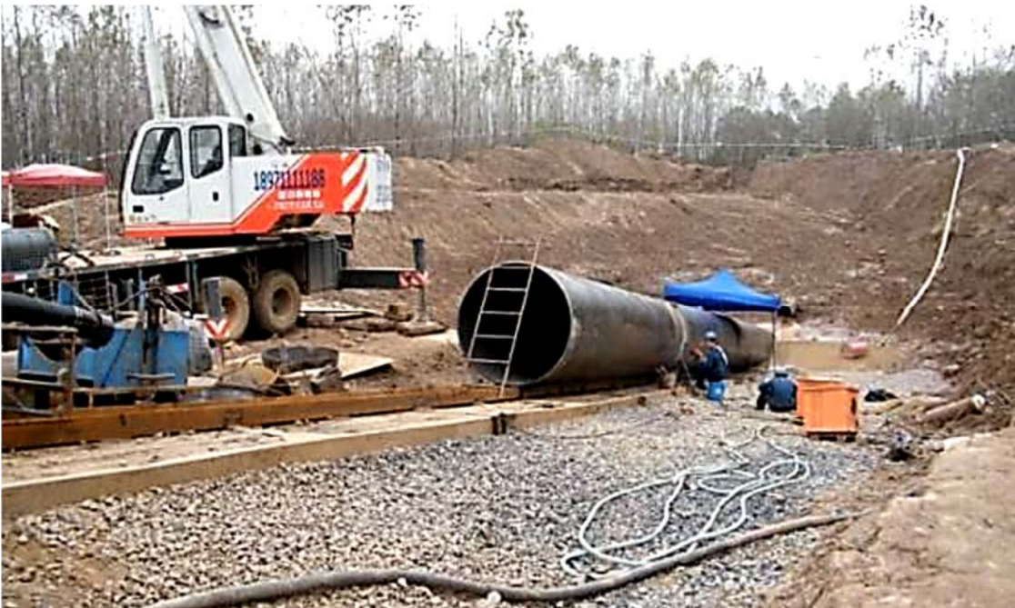
Figure 5.31: Casing Tamping Field on the North Bank (Li et al, 2013)
