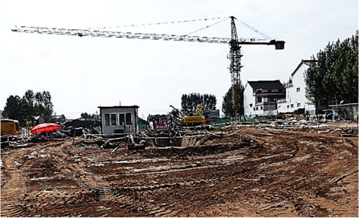
Figure 6.33: Site Overview with Safety Taping at Trench Locations
