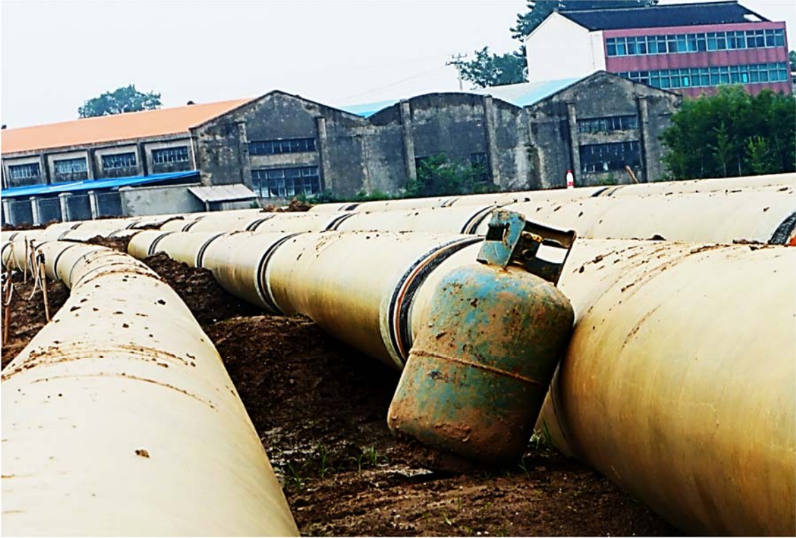
Figure 6.19: Product Staging During Welding Operations (Example 1)
