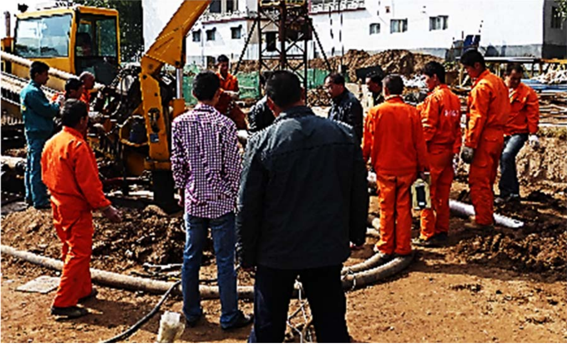
Figure 6.40: Onsite Workers During Drilling Operations
