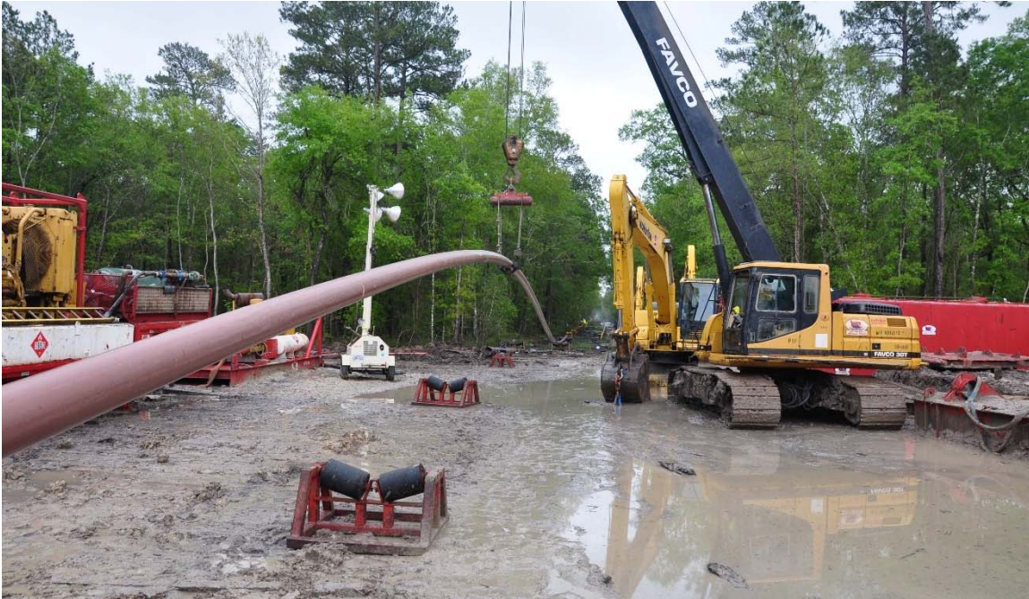
Figure 5.45: Product Pipe during Pullback (Laney 2013)
