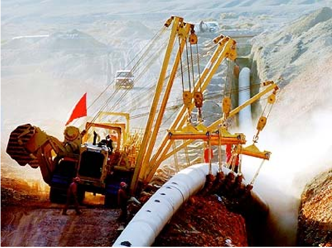
Figure 3.1: Work on the West-to-East Pipelines ( www.cnpc.com.cn/en )
