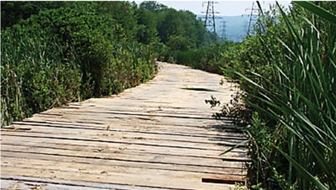
Figure 6.11: Typical Timber Matting for Site Access
