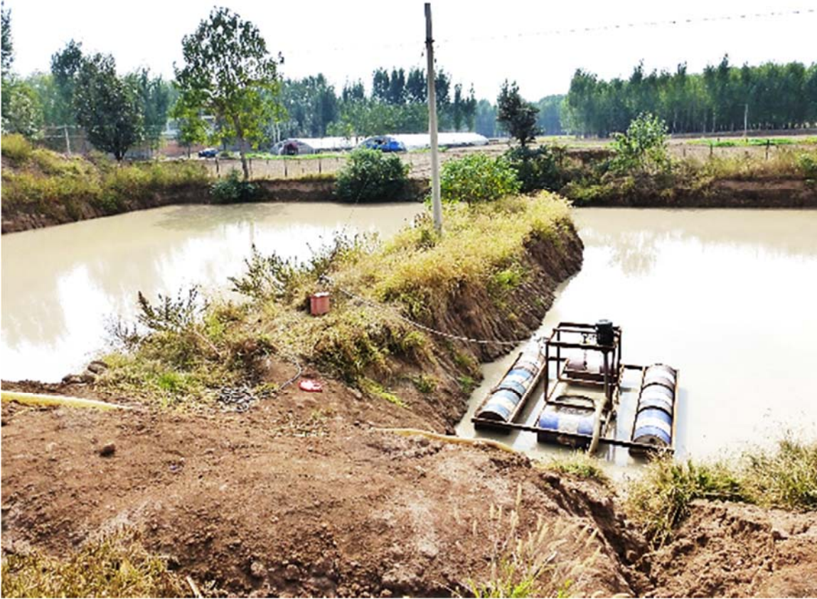
Figure 6.28: Cuttings Retention Ponding Systems (Example 2)
