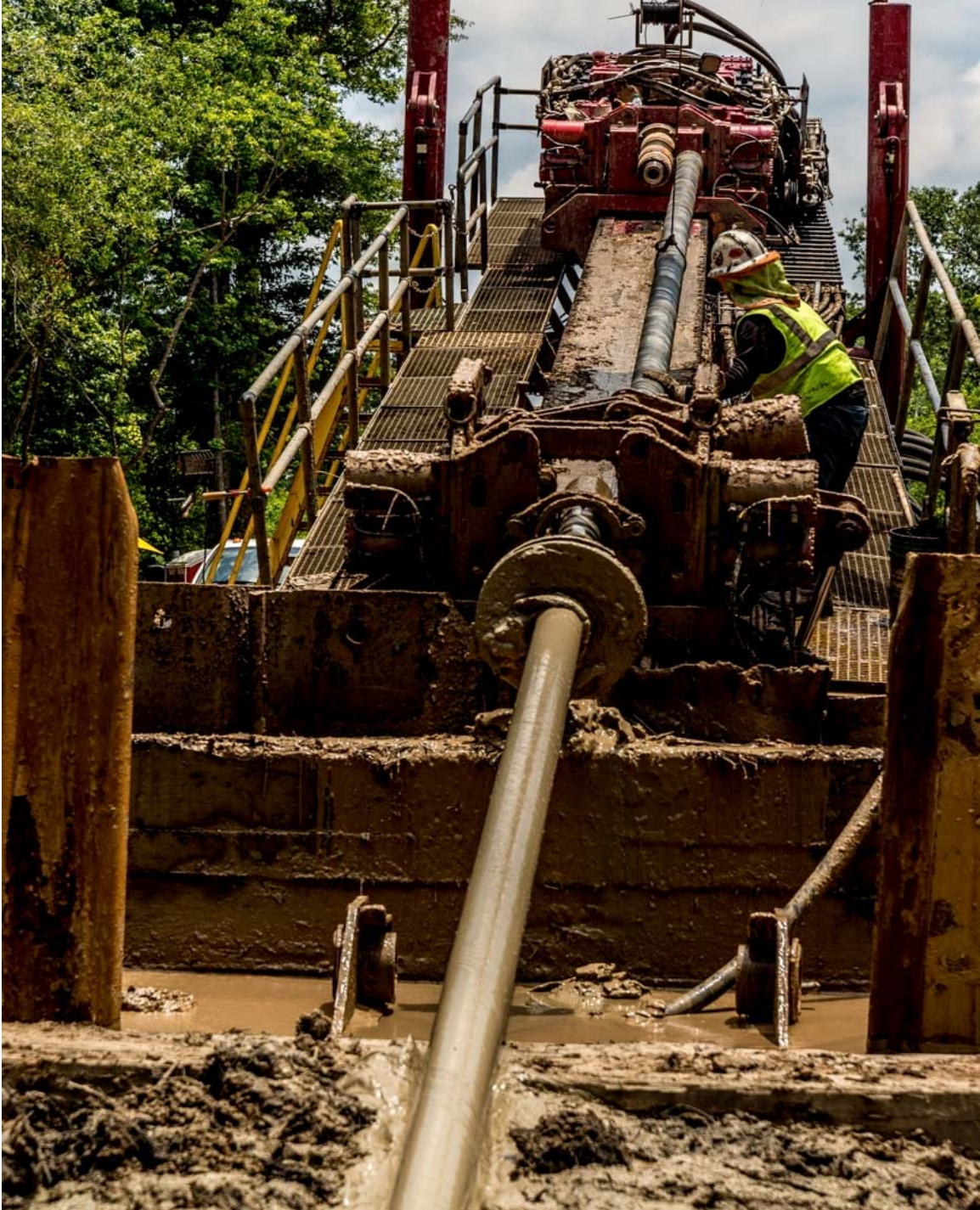
Figure 5.47: Main Drill Rig
