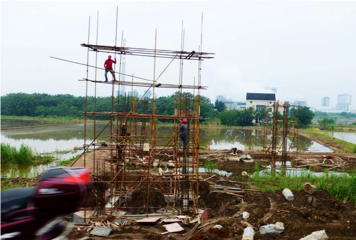
Figure 6.32: Onsite Temporary Facility Construction
