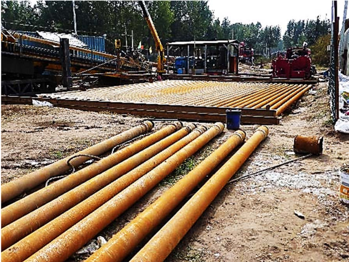
Figure 6.21: Drill Pipe – China
