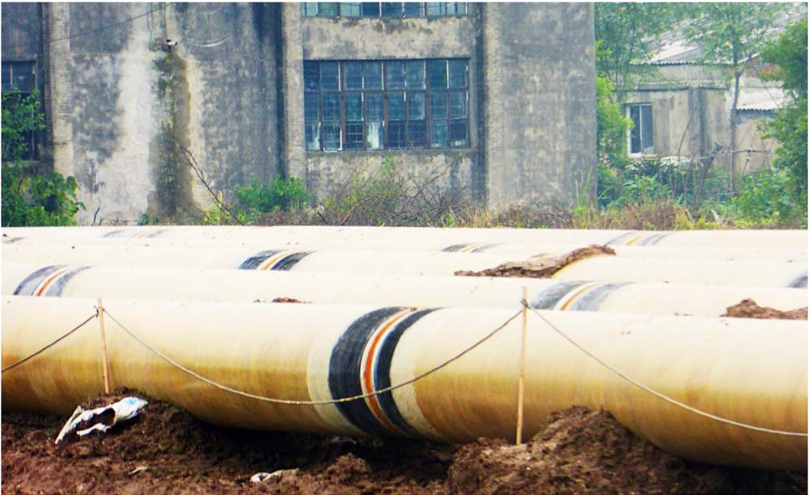
Figure 6.20: Product Staging During Welding Operations (Example 2)
