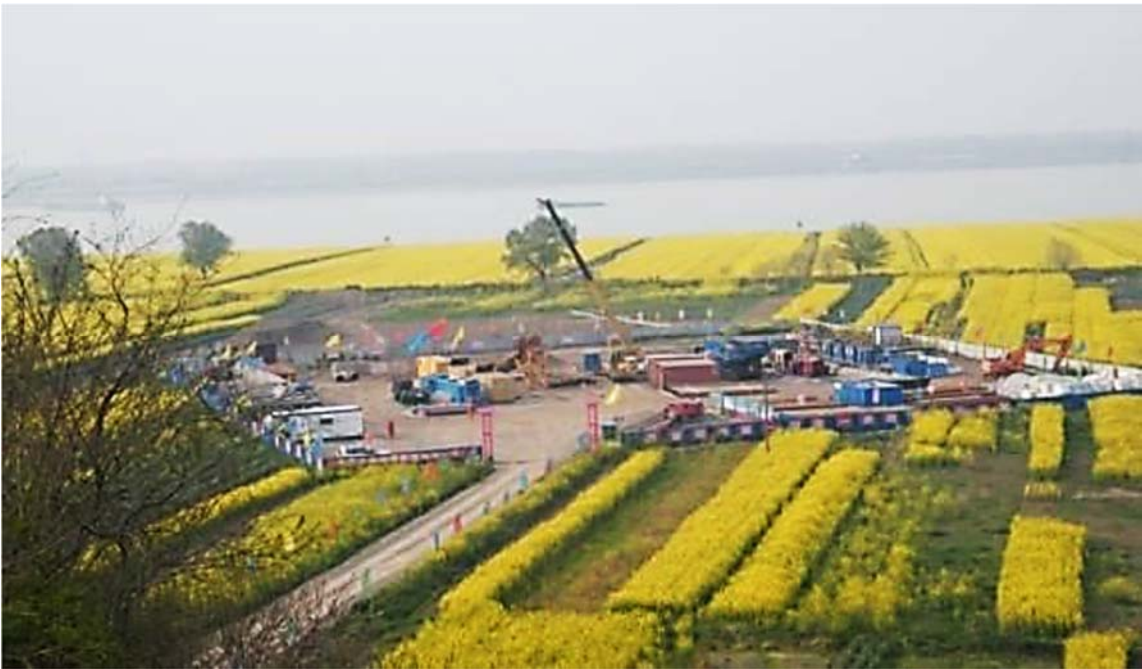
Figure 5.29: Overview of Entry Side Construction Site (Li et al, 2013)
