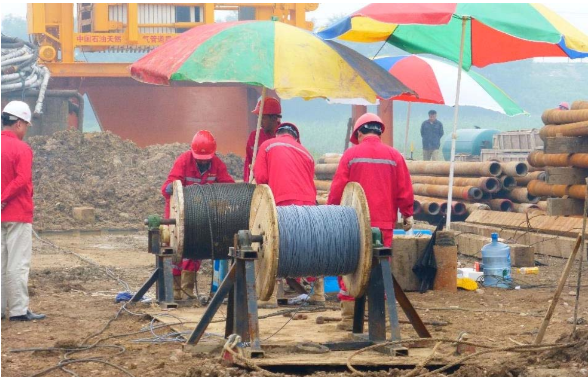
Figure 5.11: Onsite Workers Preparing ParaTrack 2 ® Tracing Lines
