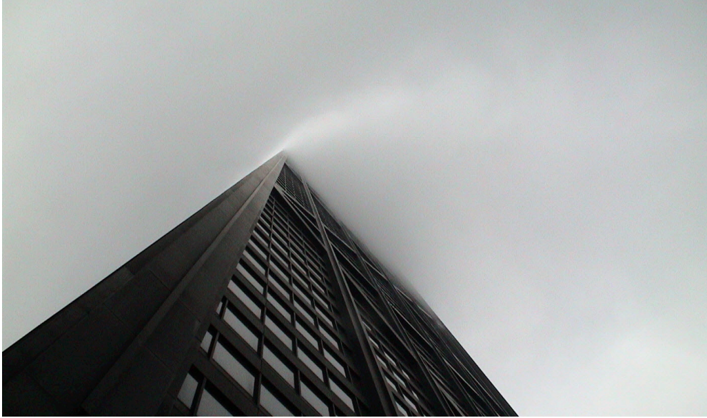
Figure 1.1.1 Vortex Shedding on John Hancock Center
