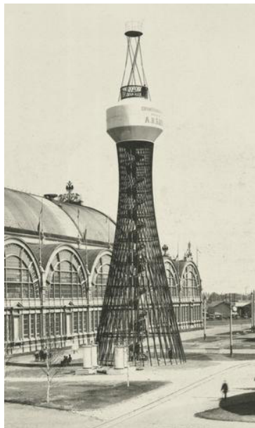
Figure 3.1.2 The World's First Diagrid Hyperboloid 37-meter Water Tower
