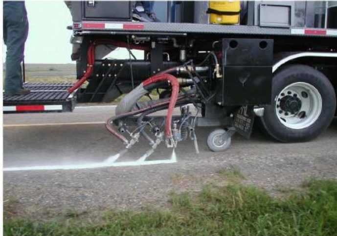
Figure 2-7: Striping Vehicle Applying Glass Beads with Spray Nozzles [14]
