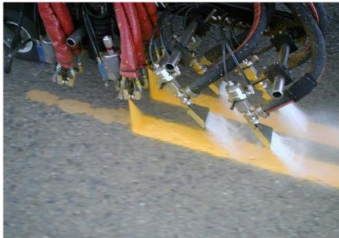
Figure 2-8: Application of Striping and Glass Beads Over Existing Marking [14]
