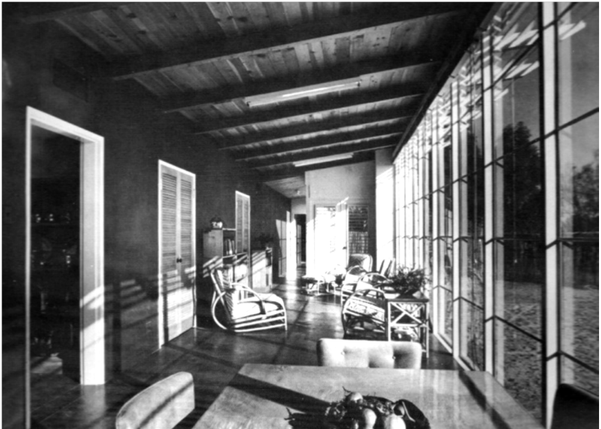
Figure 3: Internal faces of corridor walls painted black to re-radiate the solar gains. Rosenberg Residence, Tucson, Arizona.
