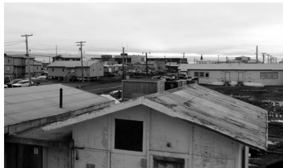
Fig. 11. View across the rooftops of downtown Barrow, AK. 2012.
