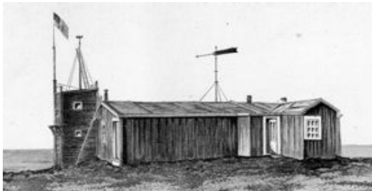
Fig. 269. Detail of “Front View of Main Building, United States Signal Station, Point Barrow, Alaska.” Painting by John Murdoch (from Murdoch 1988:frontispiece).
