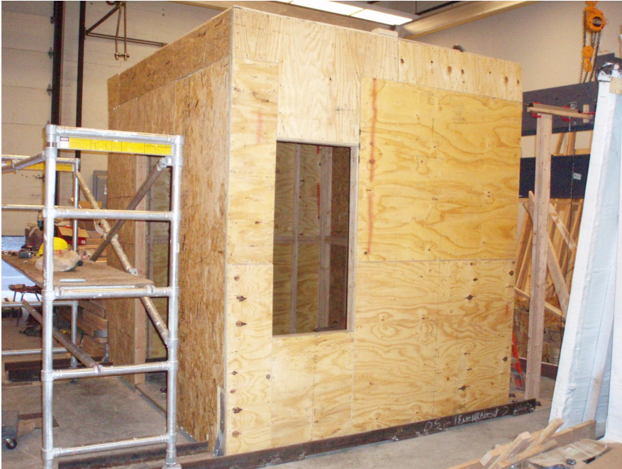
Figure 27. The single-story wood structure.
