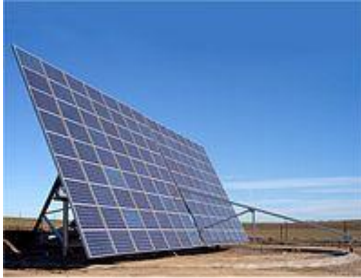
Fig 3.20 Azimuth-Altitude Dual Axis Tracker
