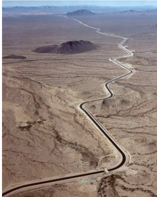
Figure 6 Central Arizona Project Canal
