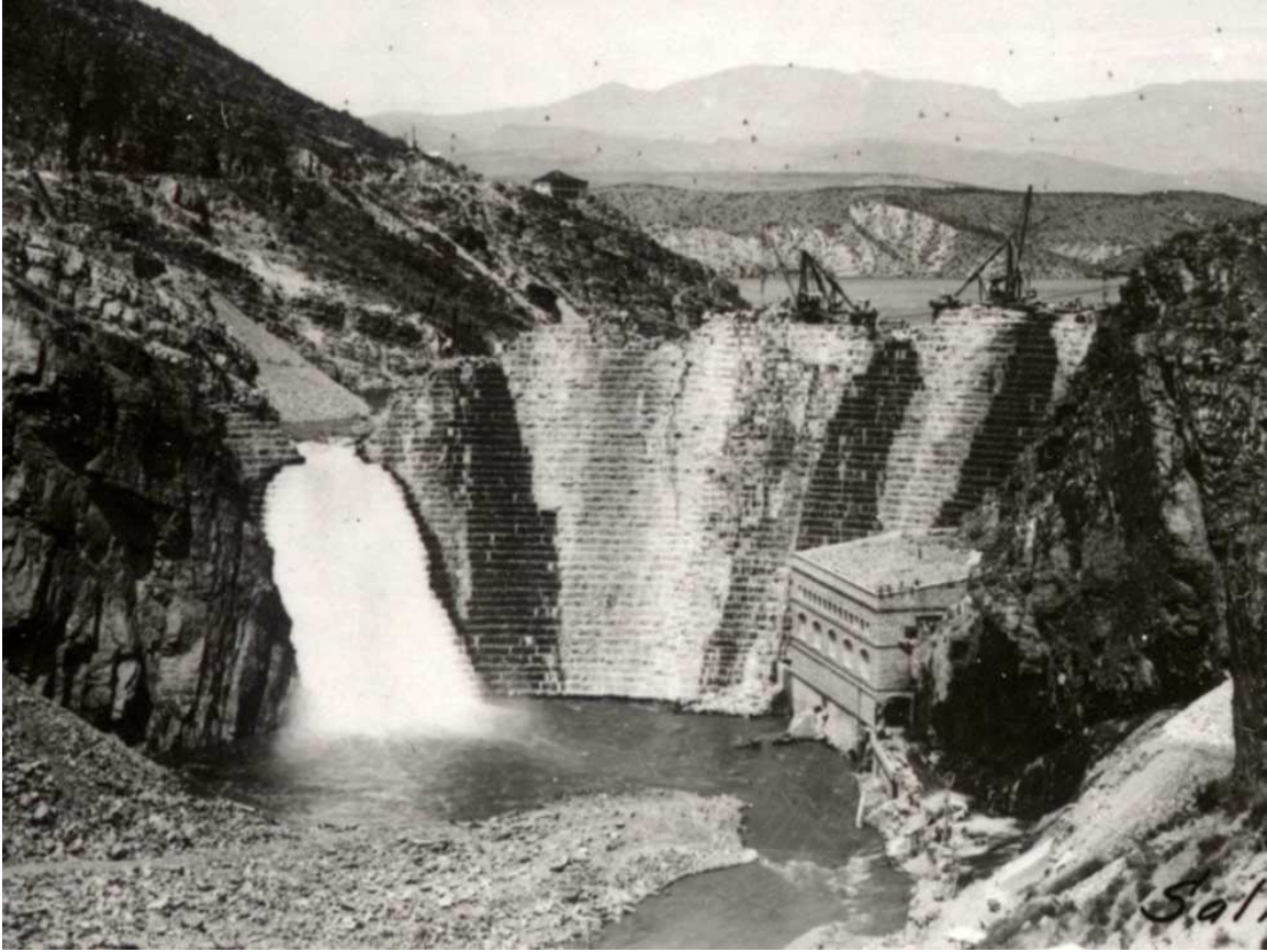
Figure 3 Roosevelt Dam under construction
