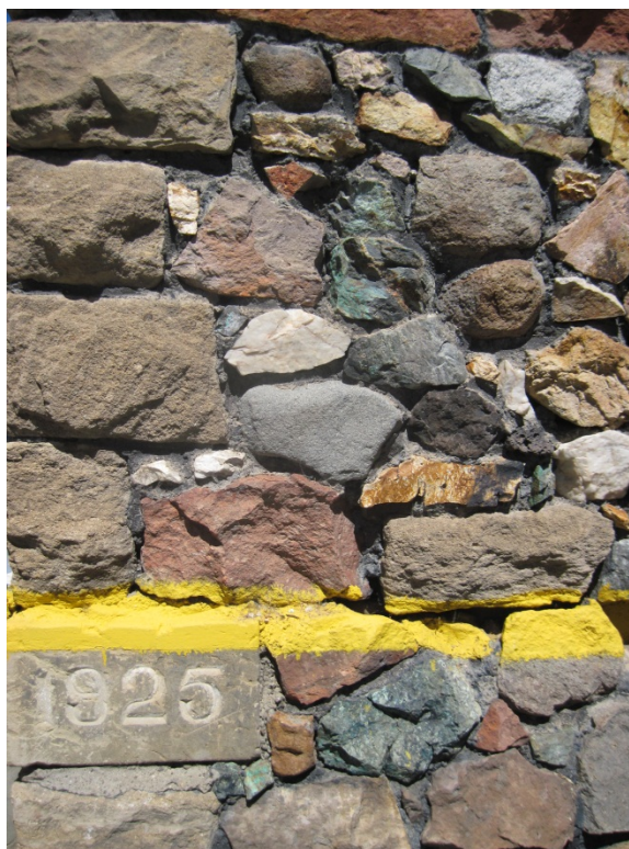
Figure 10: Stonework on the Stewart post office. The distinctive Stewart architectural style has randomly shaped native stones set in dark mortar. Rectangular corner stones on the left are common on the campus buildings. Photograph taken by the author May 21, 2010.
