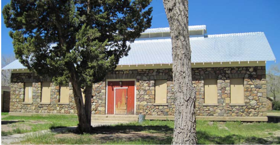
Figure 11. The band building demonstrates the varied colors of native stone and dark mortar used in Stewart architecture. Photograph taken by the author May 21, 2010.
