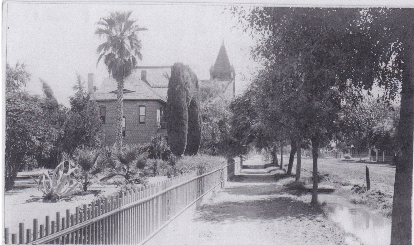
Figure 4.4: Water from acequias fed shading vegetation in wealthy neighborhoods in central Phoenix. Barry M. Goldwater Historic Photograph Collection (FP FPC 1, Box 8, Folder 1. Historic Photographs, Places: Canals and Irrigation. 1890-1901. Arizona Collection, Arizona State University Libraries.
