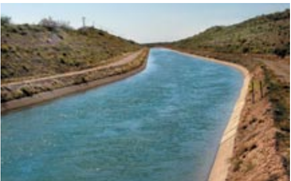
Central Arizona Project, near Florence
