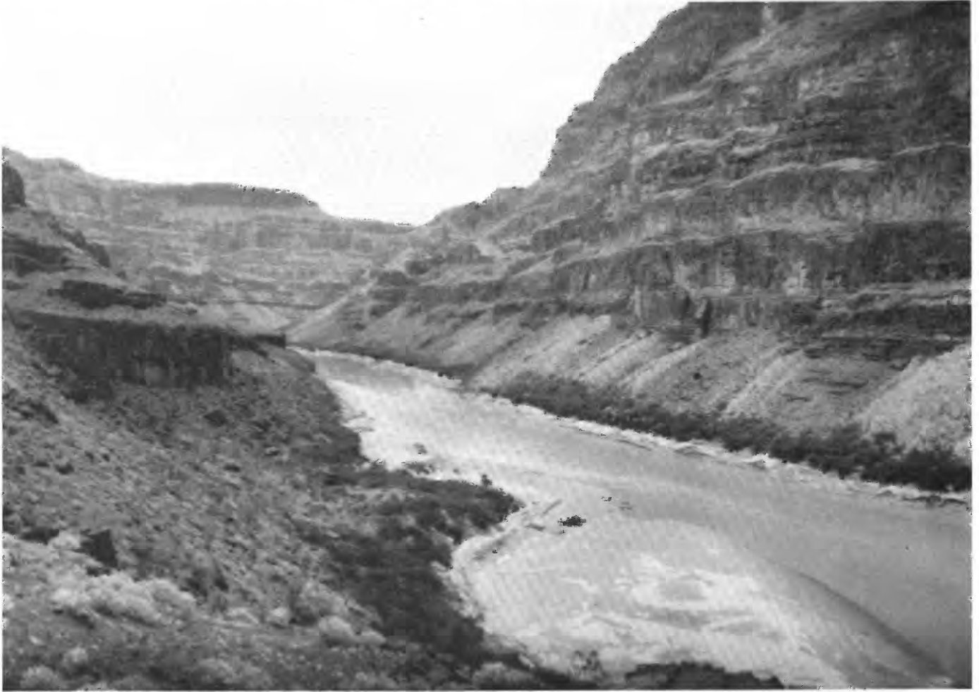
FIGURE 61A.—(1923). This upstream view was taken from a point just above Spring Canyon, 328.9 kilometers below Lees Ferry. The Middle Cambrian Bright Angel Shale, mostly covered by slope wash, is at river level. A well-developed community occurs above the flood line on both sides of the river. At the present river stage, a large bar, unoccupied by plants, is exposed. (Altitude 454 meters.)
