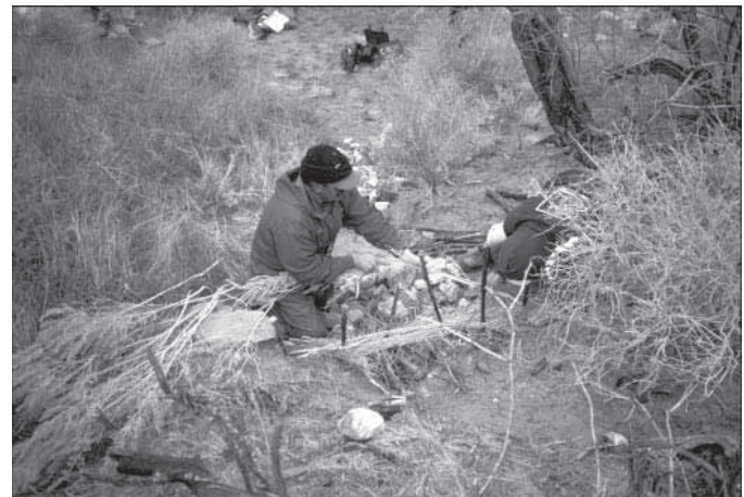
Figure 6. Members of the Zuni Soil Conservation Project constructing a check dam by using the basket-weave technique (photograph courtesy of Grand Canyon National Park).
