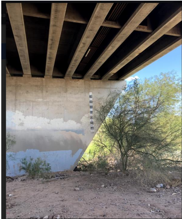
Figure 10: Central Avenue Bridge from trail
