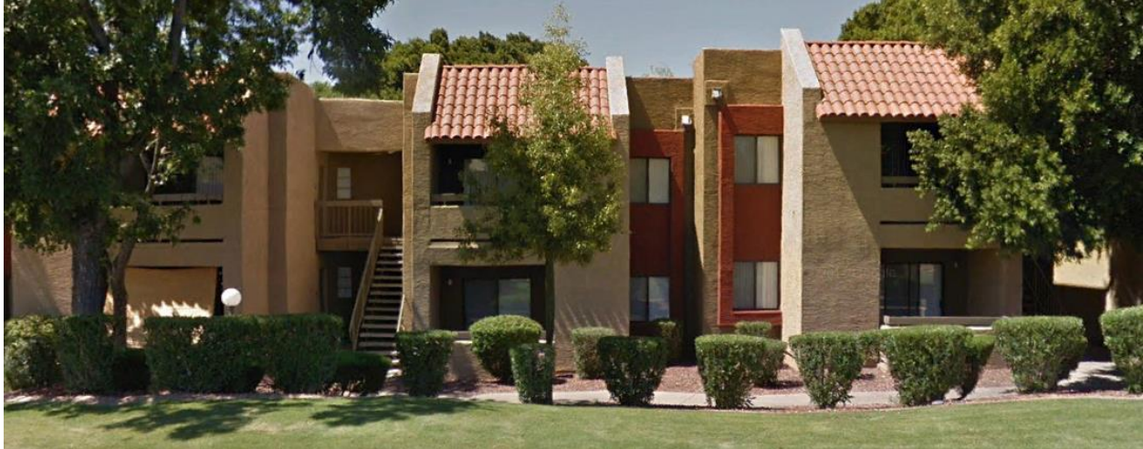
Figure 2-C: Low-rise apartment buildings
