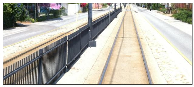
Figure 8 - At-Grade in Roadway Median Gold Line Track Segment
