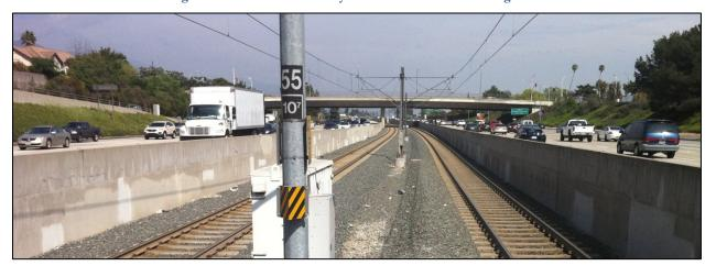
Figure 9 – At-Grade in Freeway Median Gold Line Track Segment
