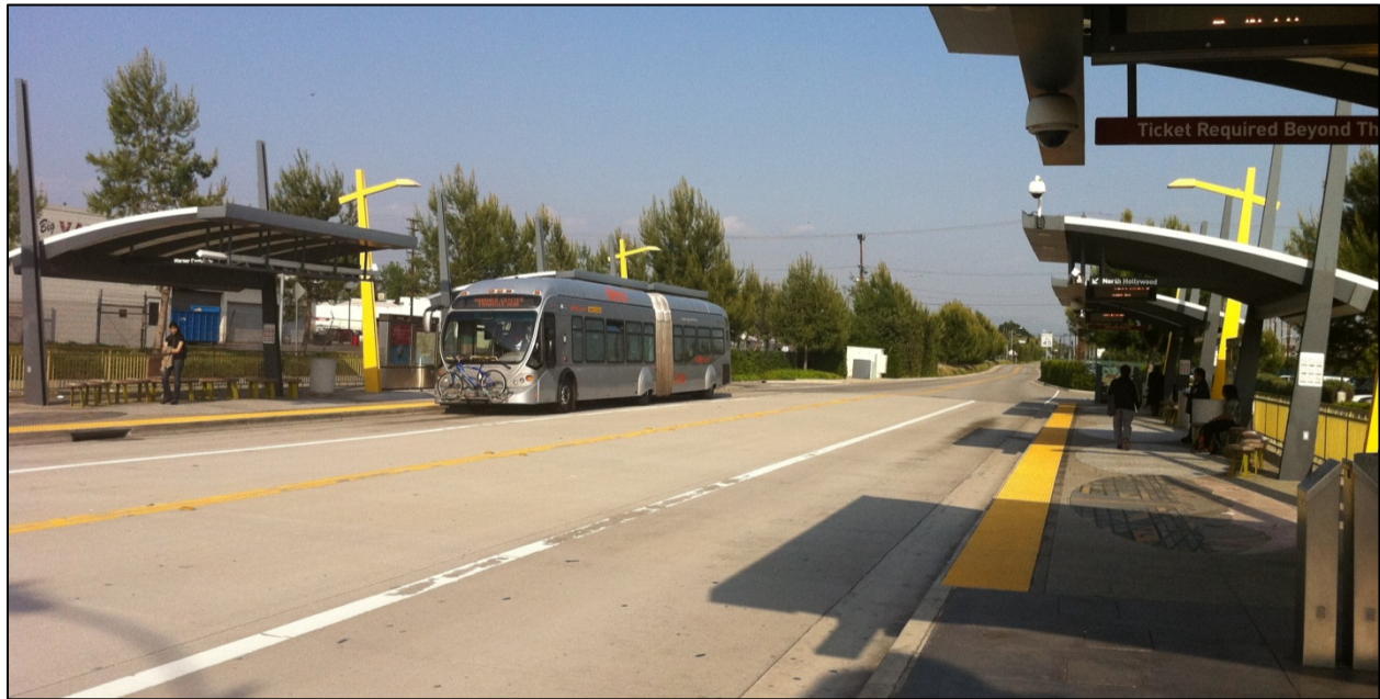
Figure 2 – Typical Orange Line Station and View of Roadway
