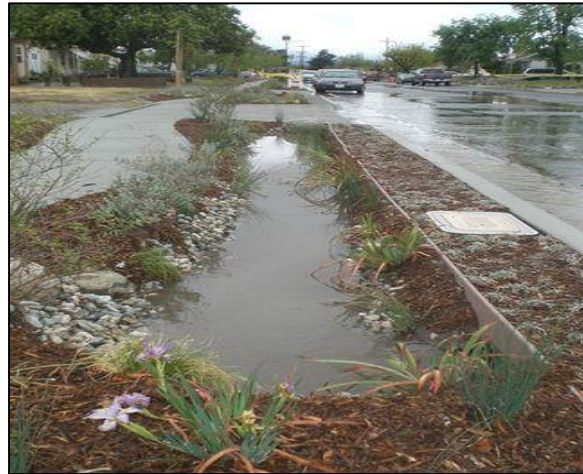
FIGURE 16. STREETSIDE BIOSWALE. PHOTO CREDIT: LOS ANGELES AND SAN GABRIEL RIVERS WATERSHED COUNCIL
