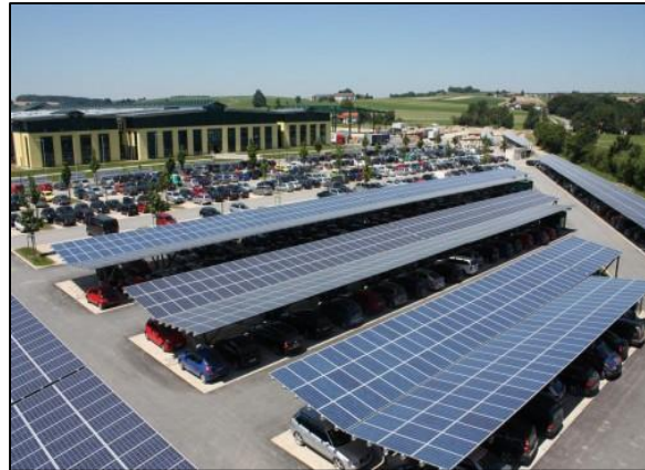
FIGURE 12. SOLAR PANEL SHADING STRUCTURE OVER PARKING LOTS. PHOTO CREDIT: CLEANTECHNICA.COM/1020/08/03/SOLAR-POWER-TRANSFORMS-PARKING-LOTS-INTO-GREEN-JOB-GENERATORS
