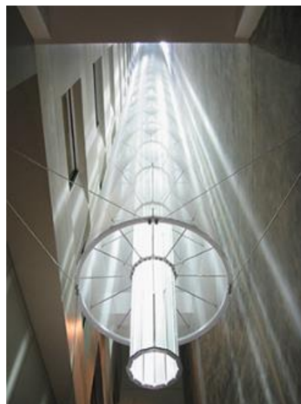
FIGURE 35. SOLAR LIGHT TUBE INSTALLED IN THE INTERNATIONAL LAW OFFICE OF MORGAN LEWIS, WASHINGTON, DC
