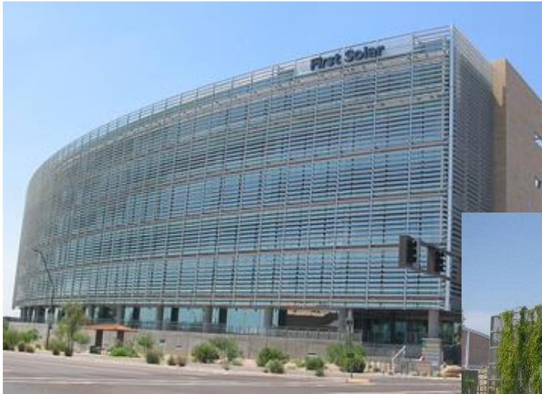
FIGURE 36. EXAMPLE OF MECHANICAL FACADE
