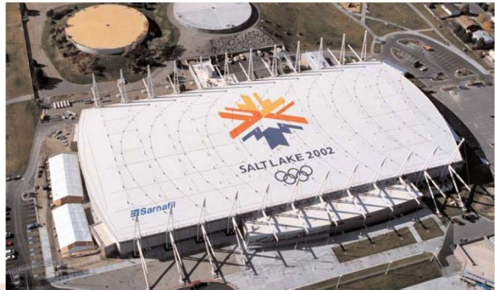
FIGURE 33. THE UTAH OLYMPIC OVAL USED COOL ROOF TECHNOLOGY
