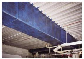
Figure 3. Steel jacketing retrofit of a beam in a building
