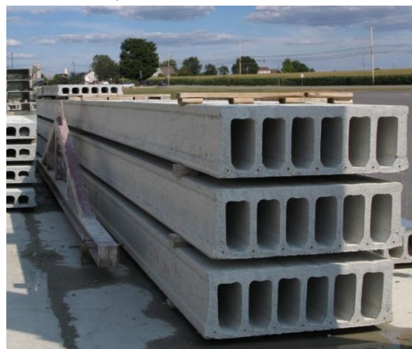
Figure 2: Pre-Cast hollow-core panels
