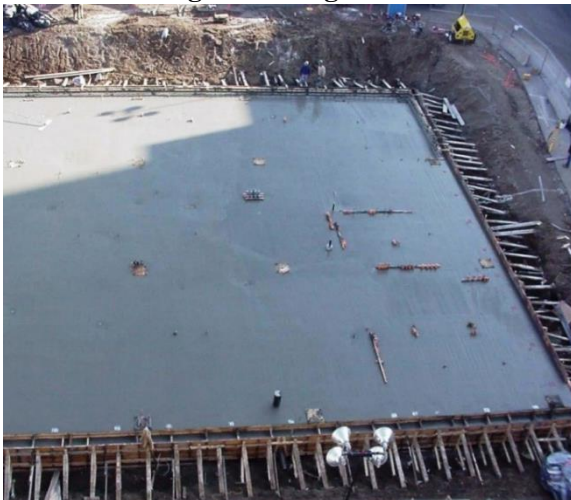
Figure 1: Cast-in-Place slab foundation
