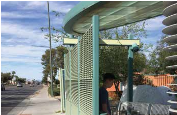
Figure 3 Perforated screen parallel with roadway provides shade on one side at all times of day. The perforation is necessary to allow views into the shaded space for security. Photo Source: Kristian Kelley
