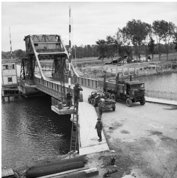
Figure 9. The Caen Canal bridge photographed on 9 June 1944 (D+3) which shows seaborne British forces using the secured bridge to move combat power inland. In the background are visible the three Horsa gliders (#91, 92, 93) in LZ “X”, with Howard’s closest to the bridge. The picture provides another excellent perspective of how the skilled landing of these gliders significantly contributed to Howard and his men achieving relative superiority and capturing this objective within five minutes. Credit: Christie (Sgt.), No 5 Army Film & Photographic Unit/ Public domain via Wikimedia Commons
