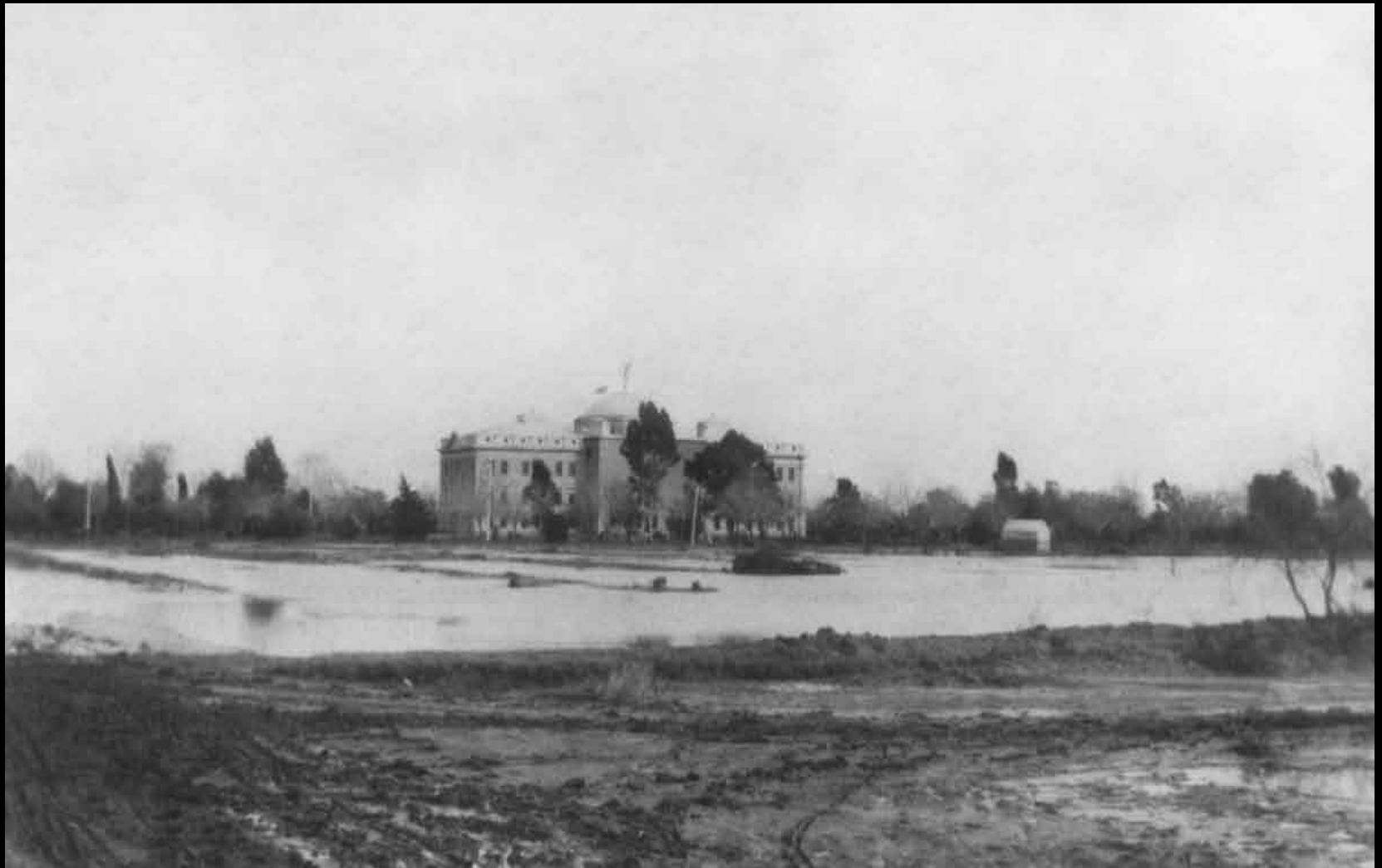
Floods reach the state capitol building
